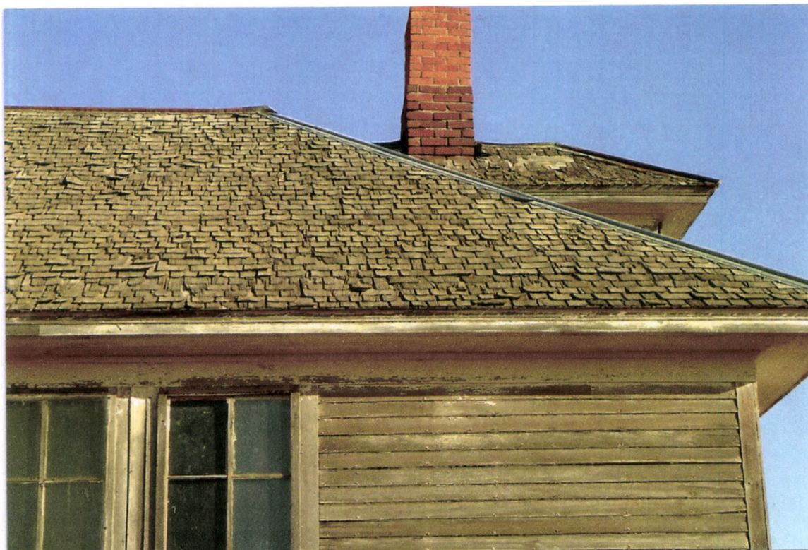
West view of roof and cupola roof and chimney.
