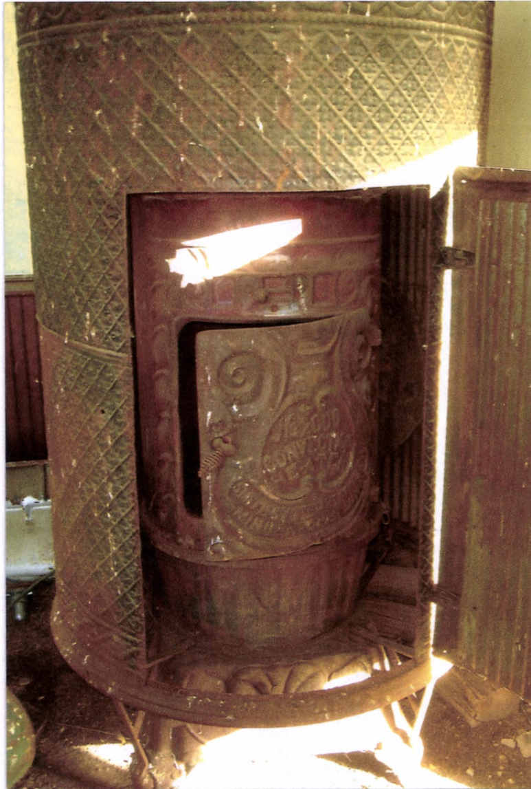
Coal/wood stove with heat shield
