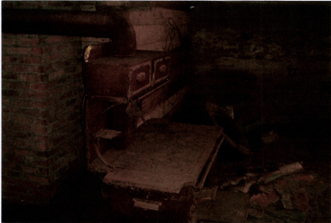
Monarch stove in basement (lower level)
