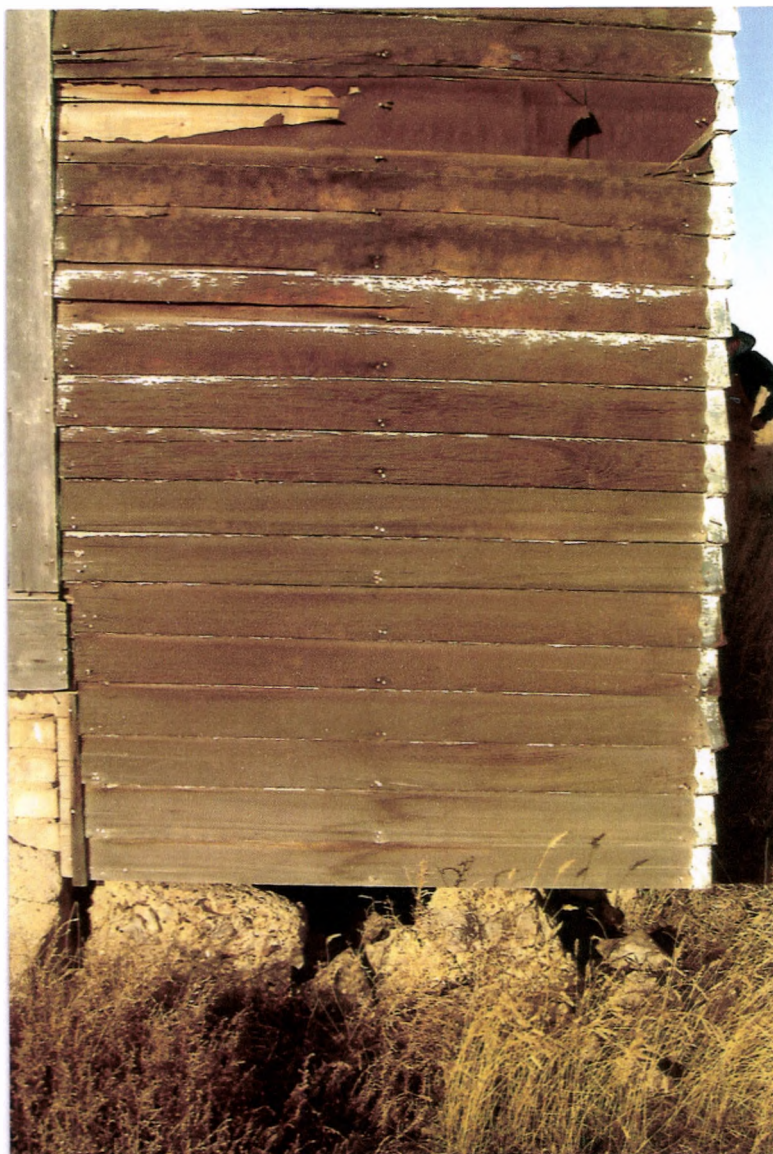
South view of lean-to built over stairway to lower level
