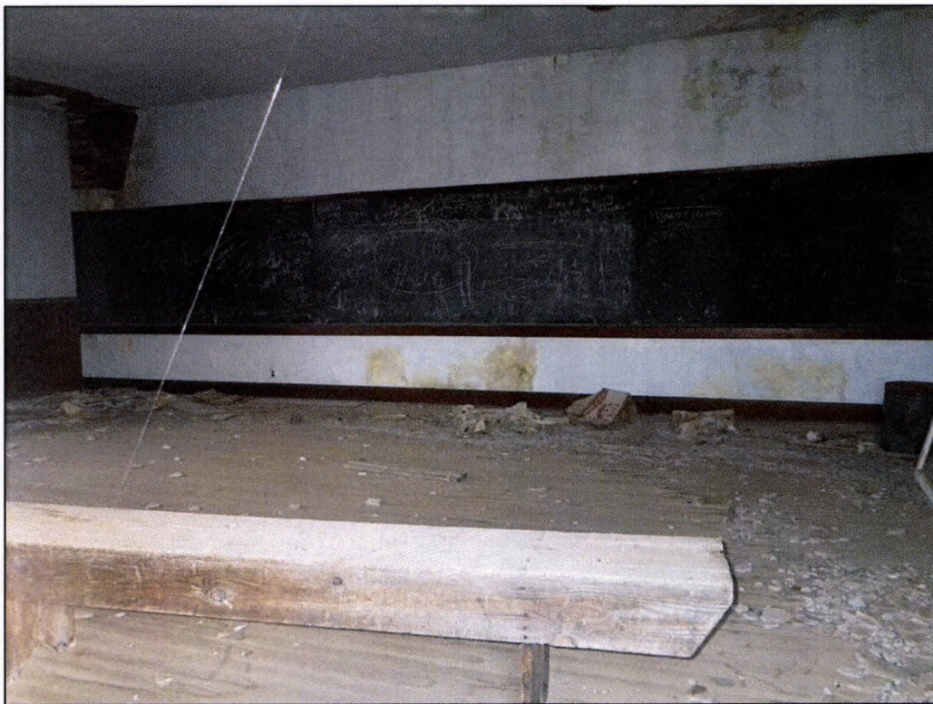
Figure 6: Feature 1, interior, view to the northwest.
