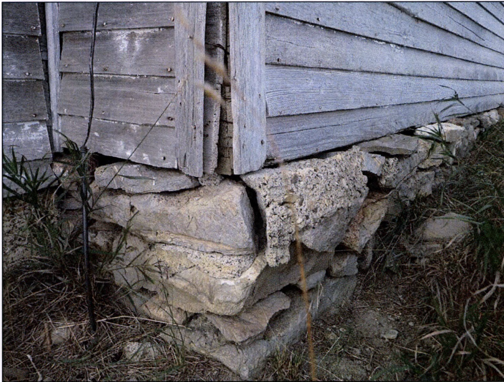
Figure 5: Feature 2, foundation, northeast corner.
