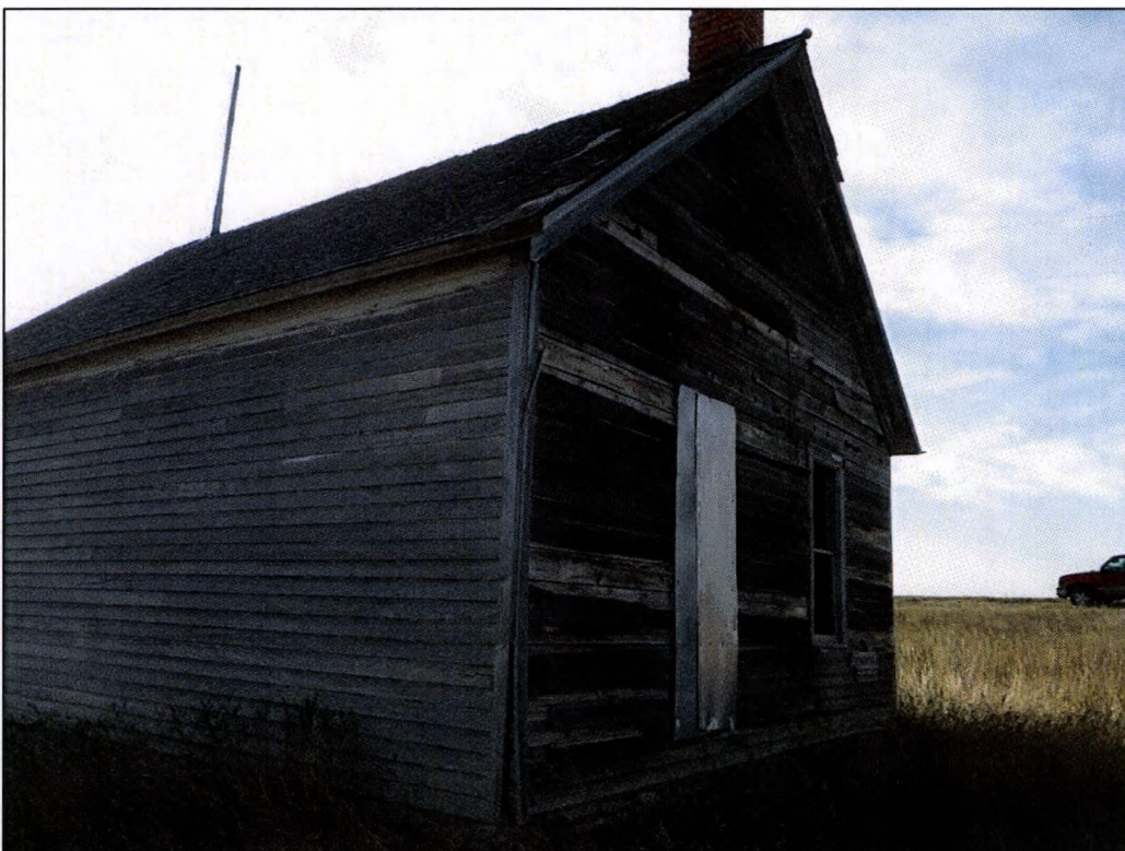
Figure 4: Feature 1, view to the southeast
