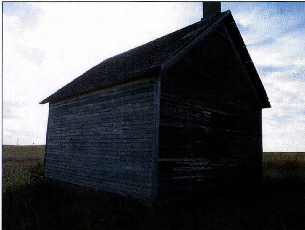
Figure 8: Feature 2, view to the southeast.
