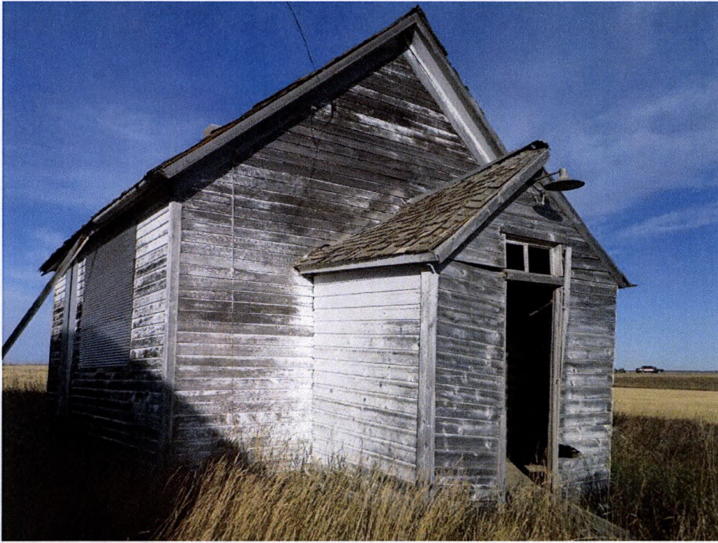
Figure 7: Feature 2, view to the northwest.
