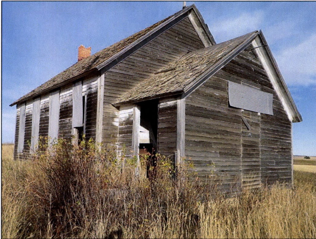
Figure 3: Feature 1, schoolhouse, view to the northwest.
