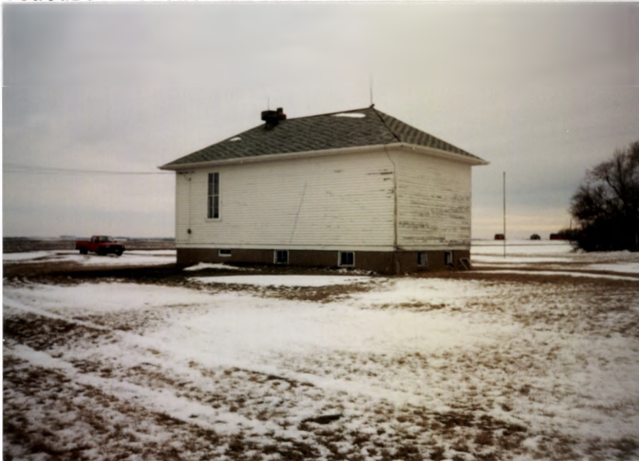
Feature 1-Rear and Side Elevation-View From NW
