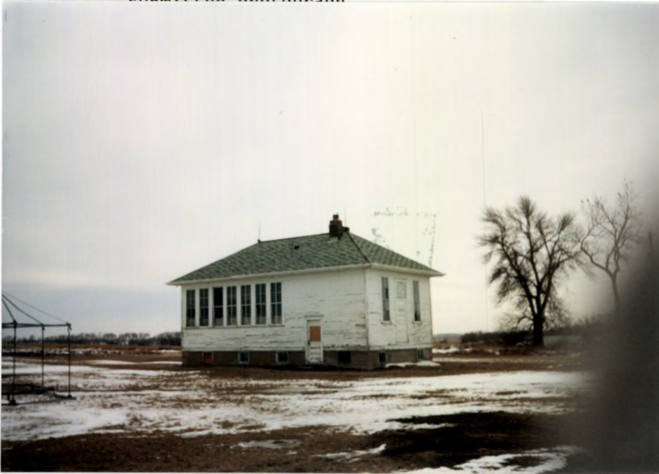
Feature 1-Front and Side Elevations-View From SE
