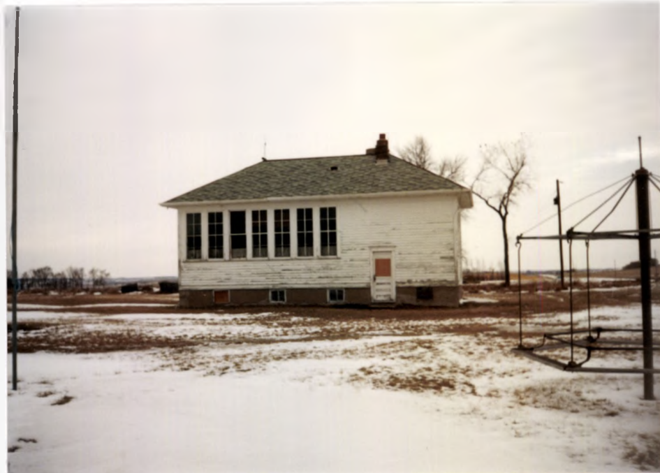
Feature 1-Side Elevation-View From South
