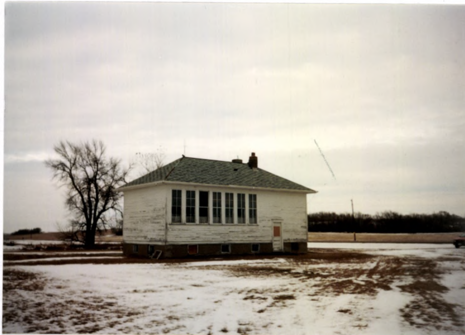
Feature 1-Rear and Side Elevations-View From SW
