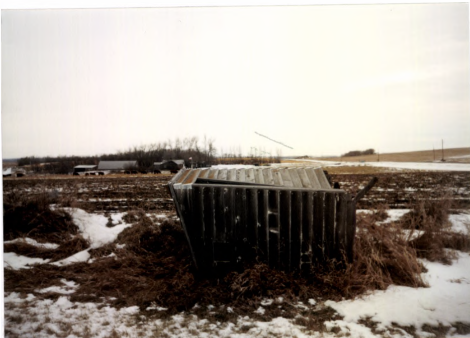
Feature 2-Privy Remains-View From South
