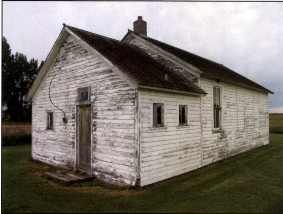
Photo 1: Northeast corner of Feature 1.
