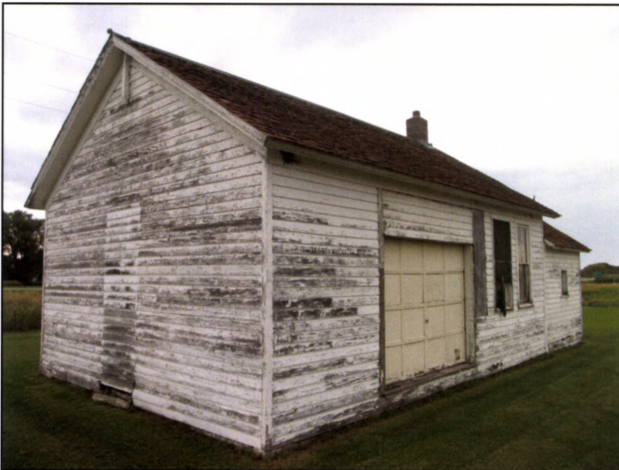
Photo 2: Southwest corner of Feature 1.
