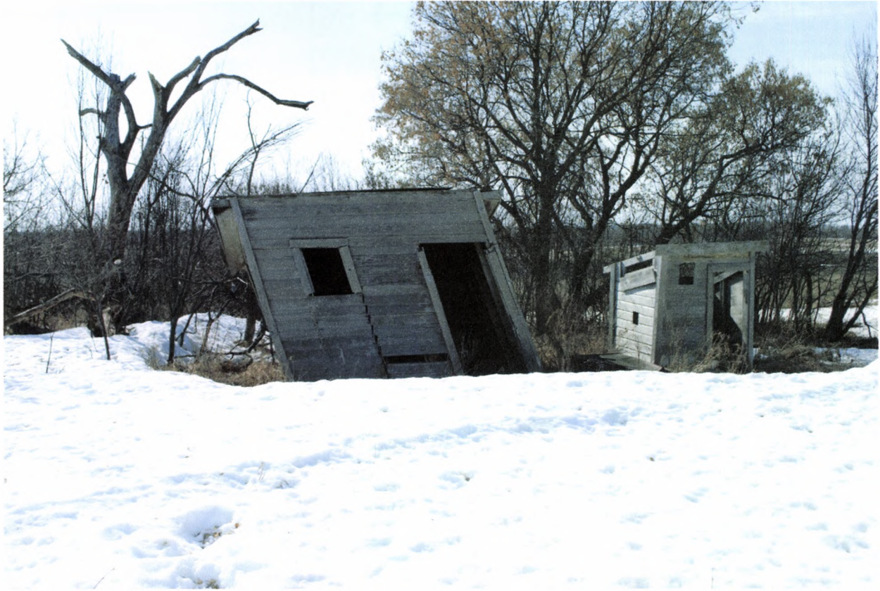
Features 2 (coal house) & 3 (outhouse) north side
