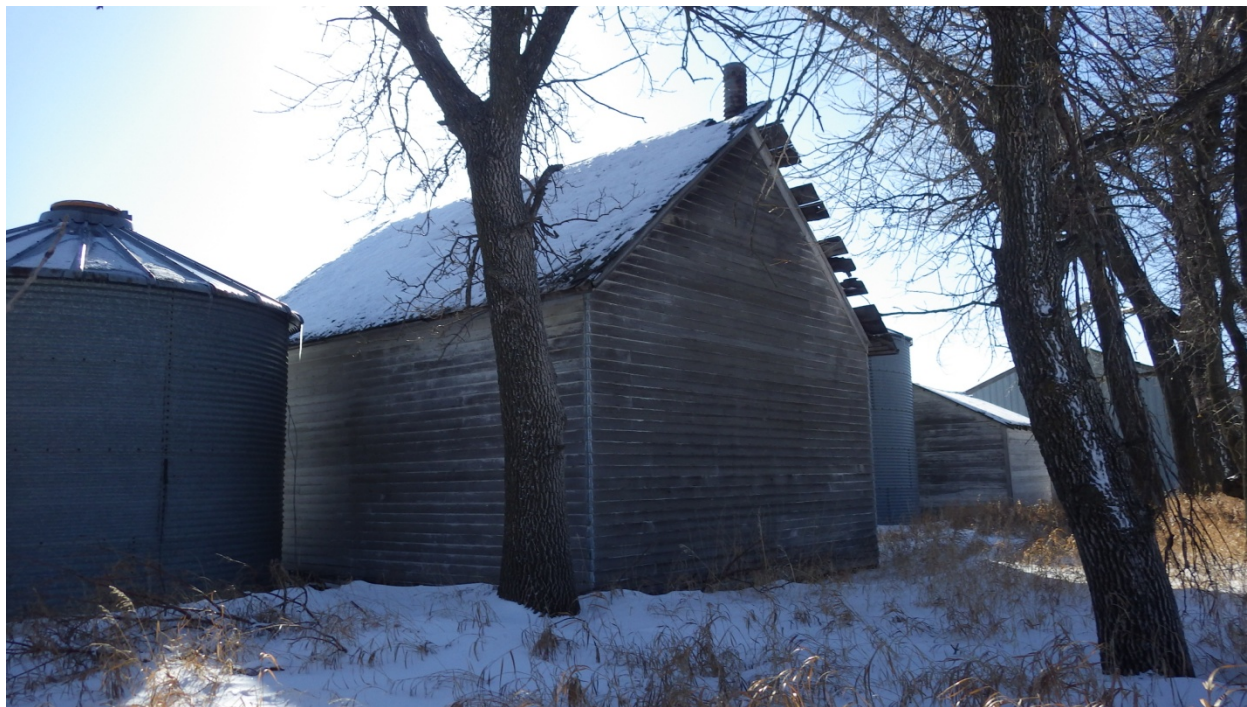
Figure 5: Site MAC-115, Feature 2, view southeast (Image 108-609).
