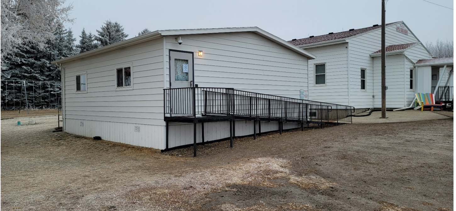
Ca. 2000 building and Feature 1 SE corner
