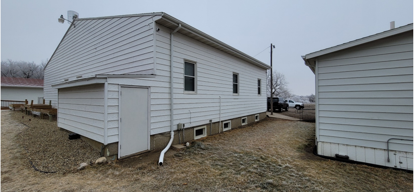
Feature 1 SW corner
