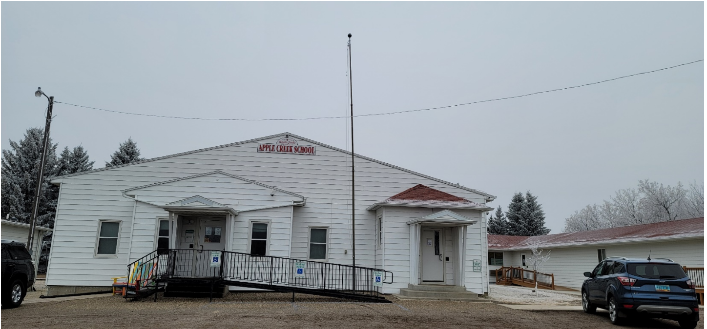
Feature 1 east façade, original school was the north portion
