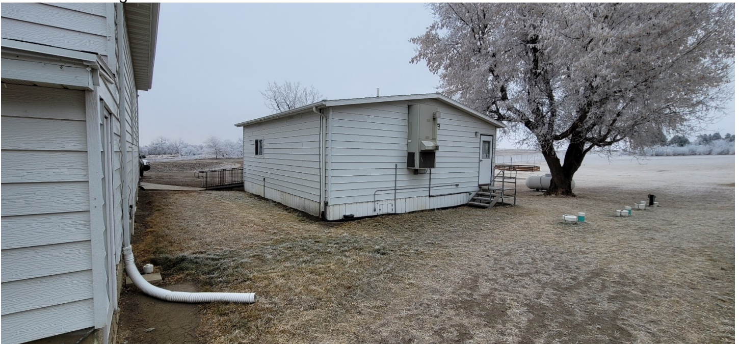
Ca. 2000 building NW corner
