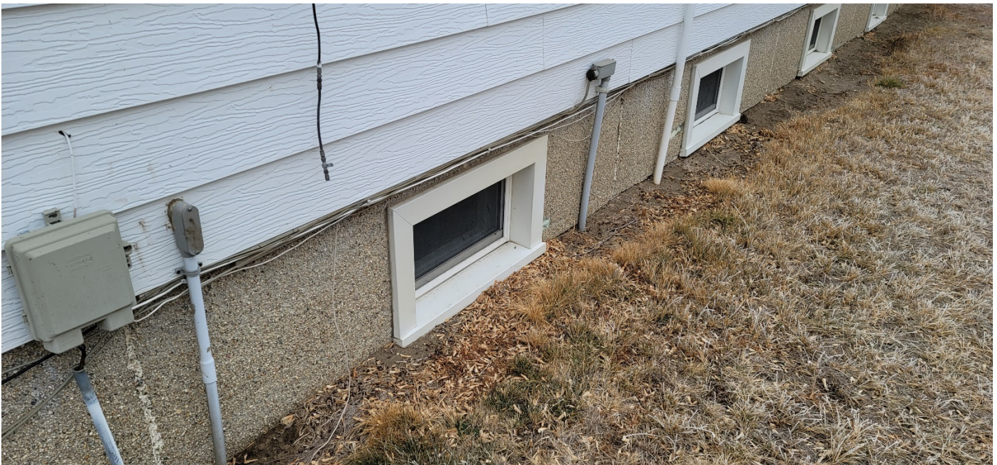
Feature 1 south side basement windows
