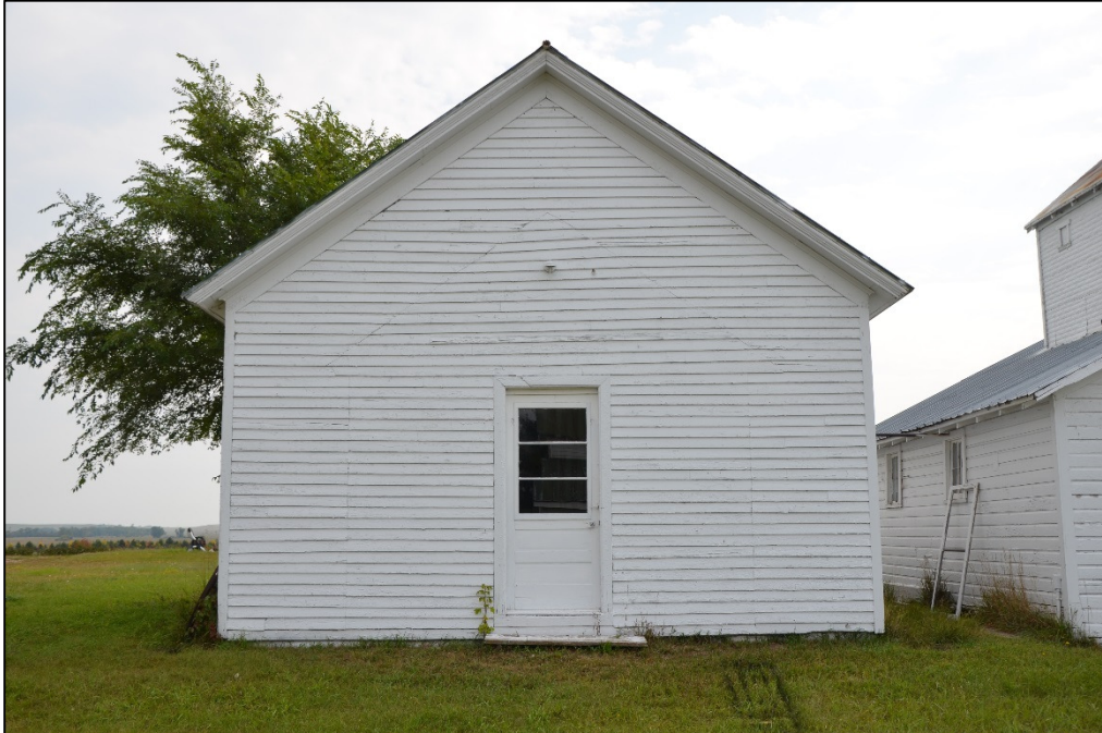
Figure 3. Feature 2, facing east (note outline of porch in paint).
