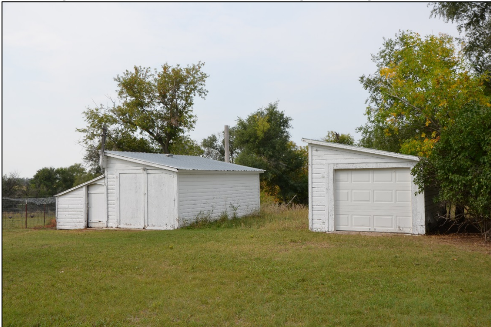
Figure 6. Features 5 and 6, facing southwest.
