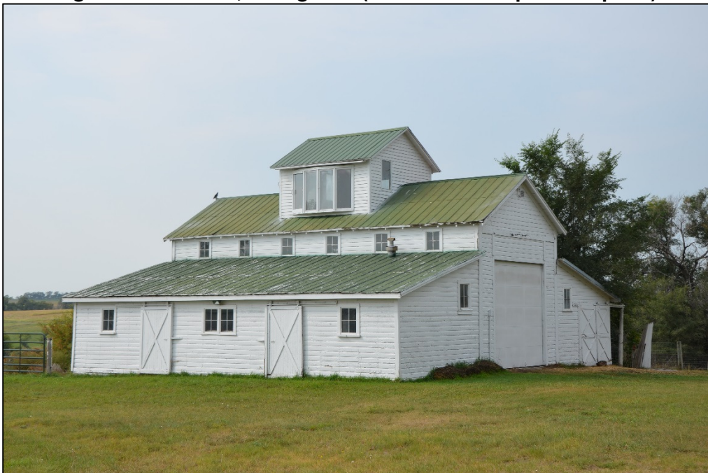
Figure 4. Feature 3, facing southwest.
