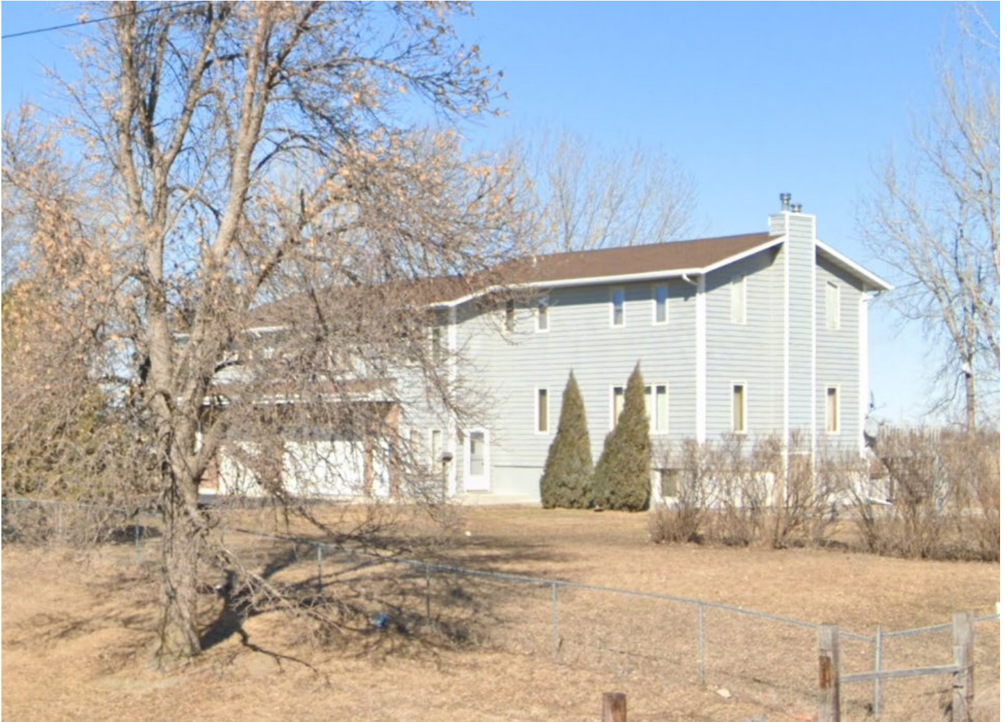
Image from Google Street View March 2022, looking northeast, showing the end that was the school.
