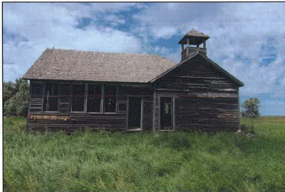
Figure 4. 32BO0163 Feature 1, Atkinson Schoolhouse facing west. M. Woods 07/26/2020.
