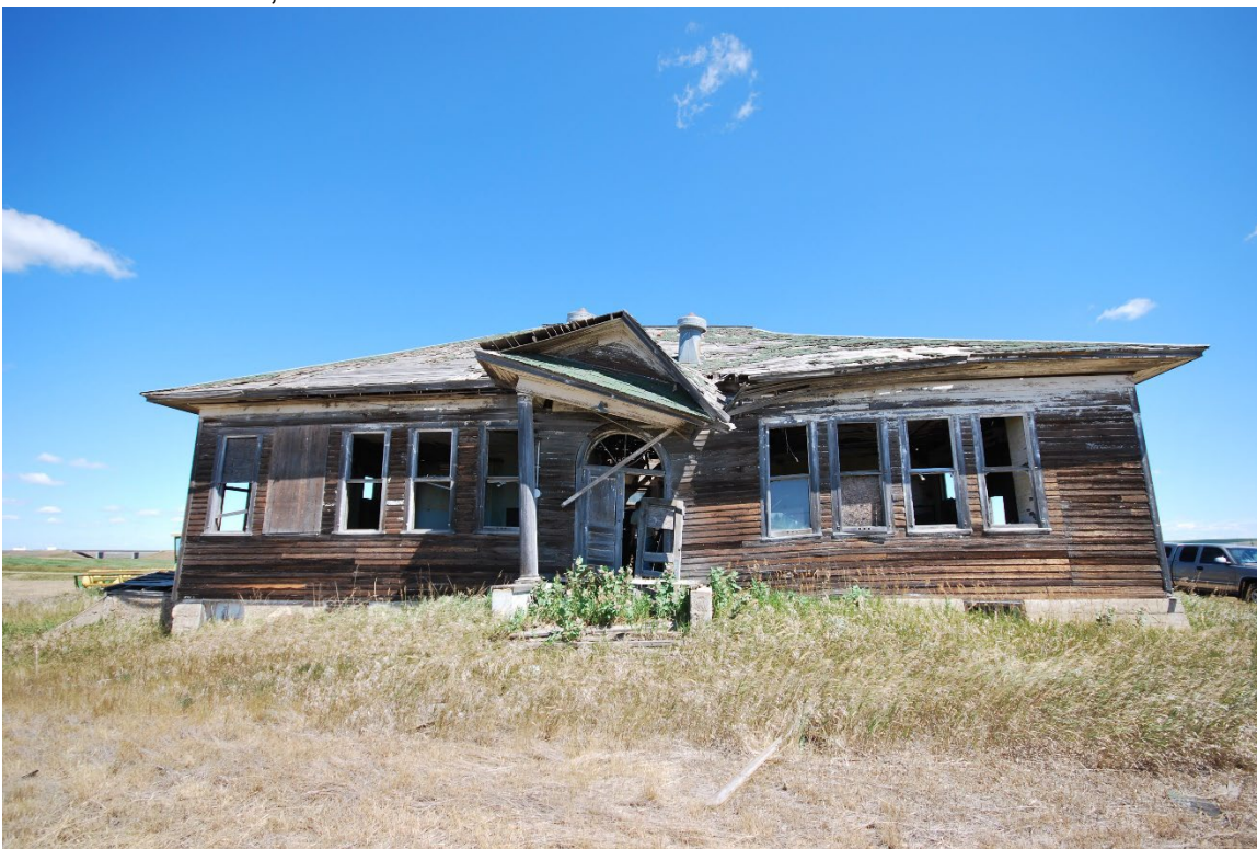
South elevation, taken 7/12/2016
