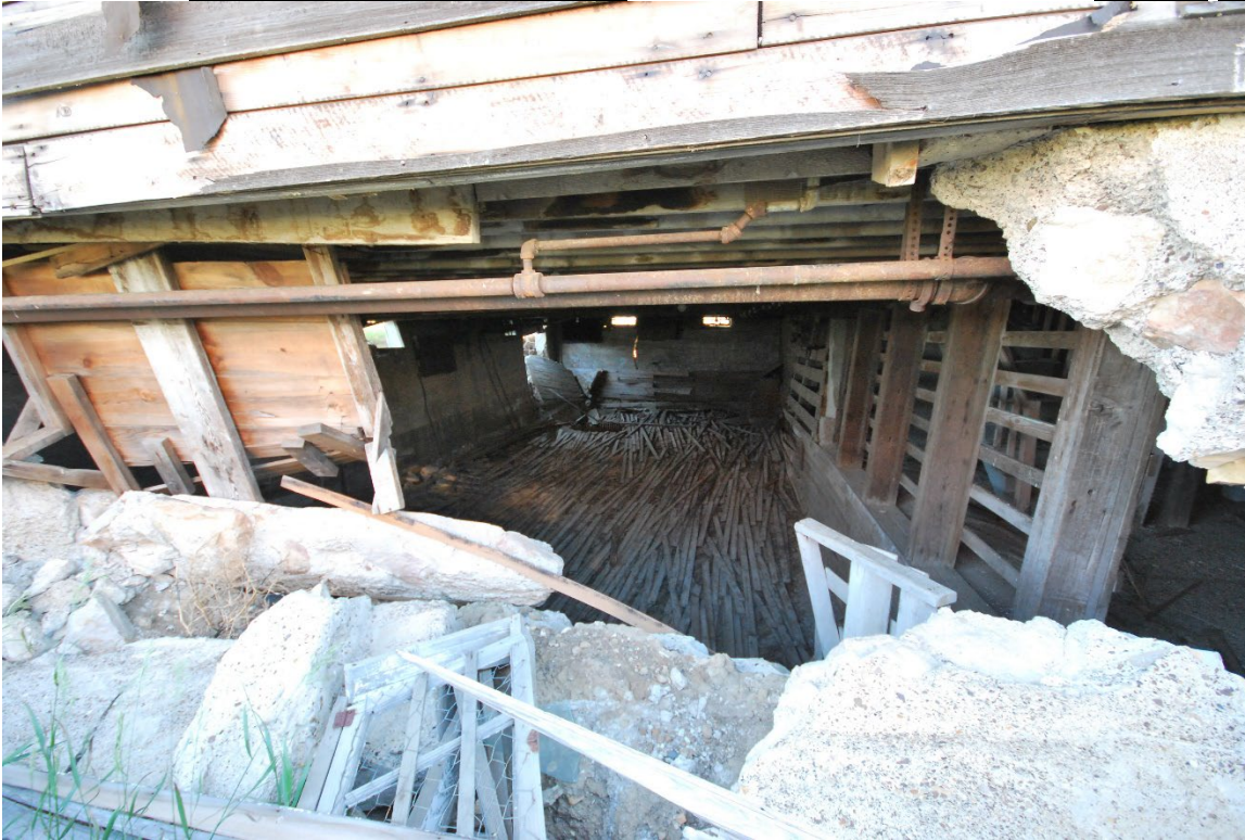
Looking into the basement, taken 7/12/2016
