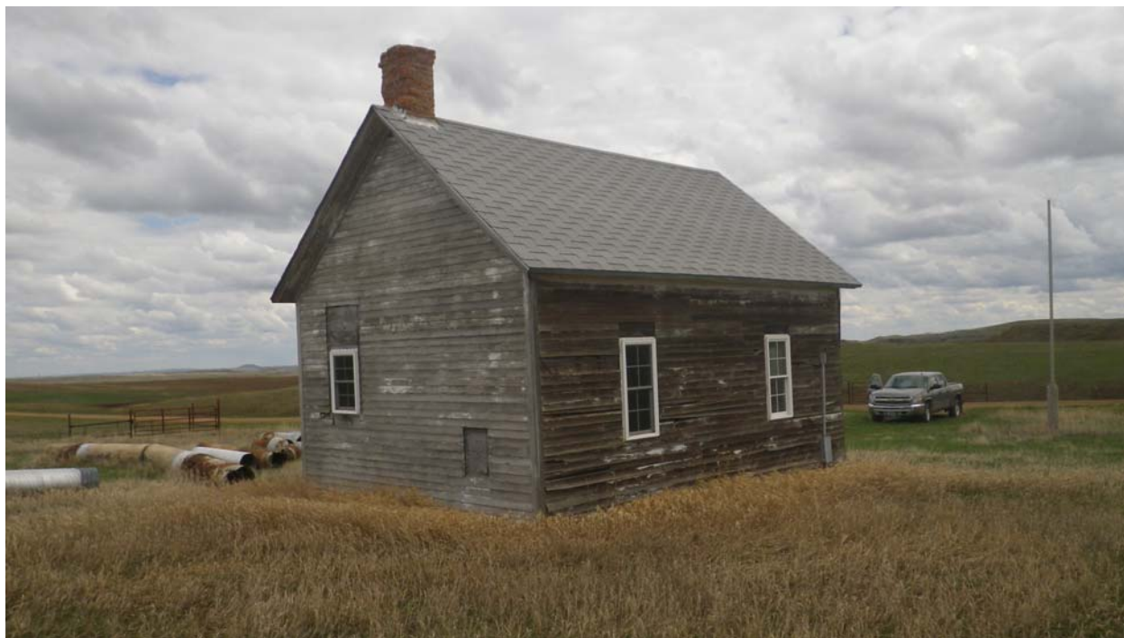
Figure 3: Site 32BO917, Feature 1 and 2, view southeast (Image 906).
