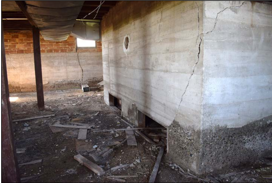
Figure 45. Ductwork and cement wall, rear of basement facing south.
