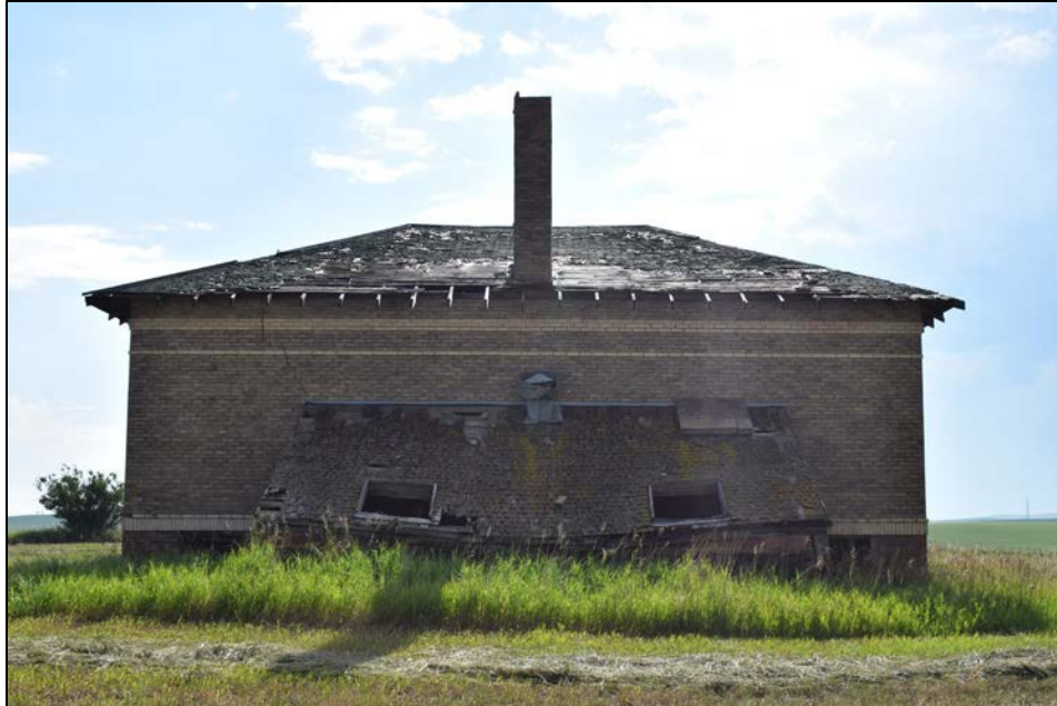
Figure 5. View of rear of QCRS-MC2A facing east.
