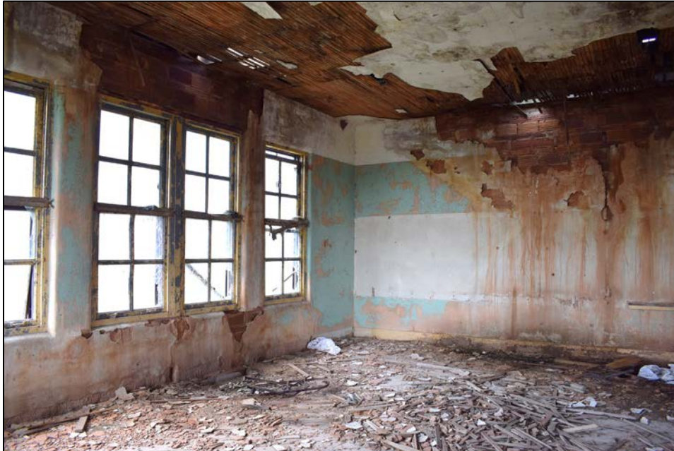
Figure 25. From south interior first floor doorway facing southwest.
