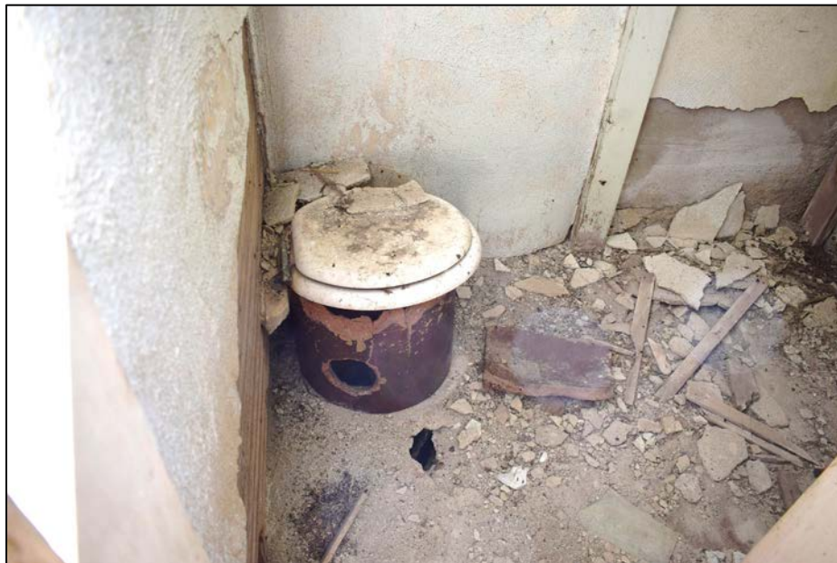
Figure 23. Girls' toilet in QCRS-MC2A facing east.
