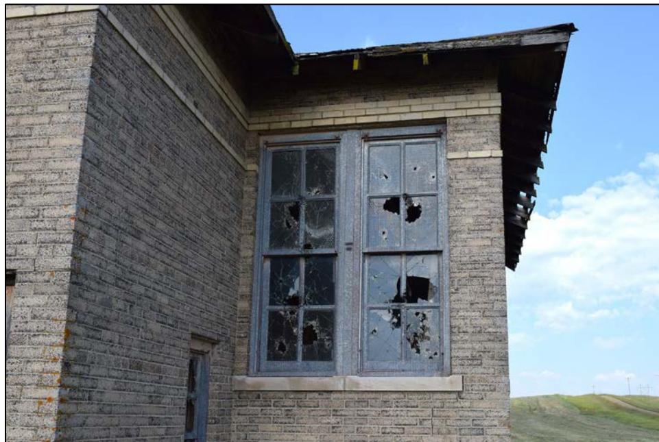
Figure 10. Additional exterior window details on front of QCRS-MC2A facing west.
