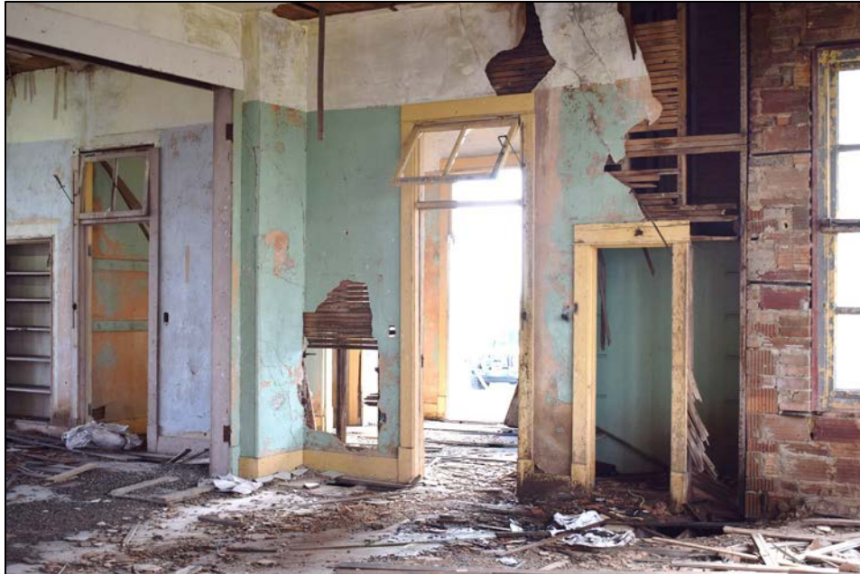
Figure 27. Southwest corner QCRS-MC2A facing northeast showing door to vestibule and exit.
