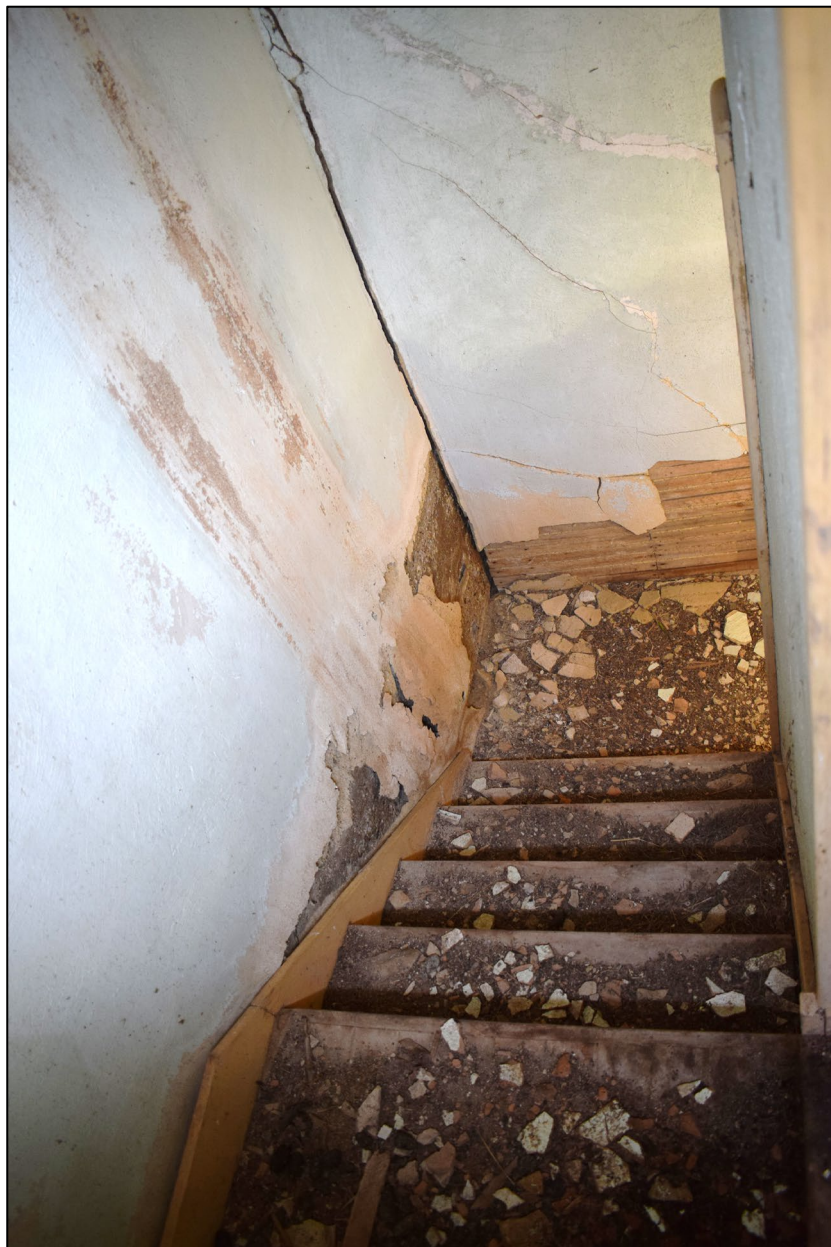
Figure 22. Stairway in southeast corner of QCRS-MC2A towards girls' toilet, directed west.
