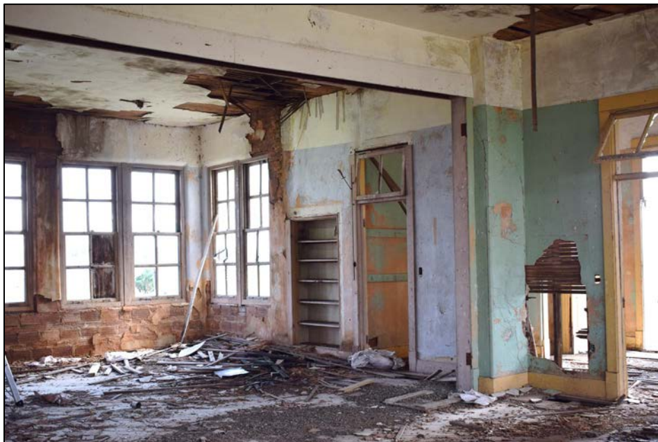
Figure 26. Interior QCRS-MC2A southwest corner facing northeast.
