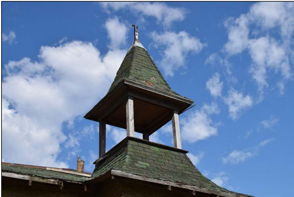
Figure 14. Detail of bell tower on QCRS-MC2A facing northwest.
