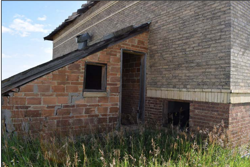
Figure 13. Detail of addition on rear of QCRS-MC2A facing northeast.
