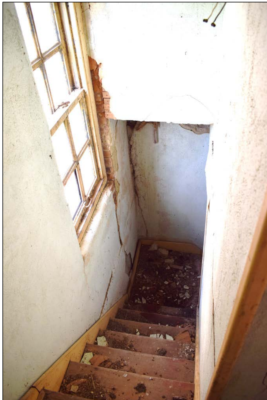
Figure 21. Stairway in south corner of QCRS-MC2A to girls' toilet facing south.
