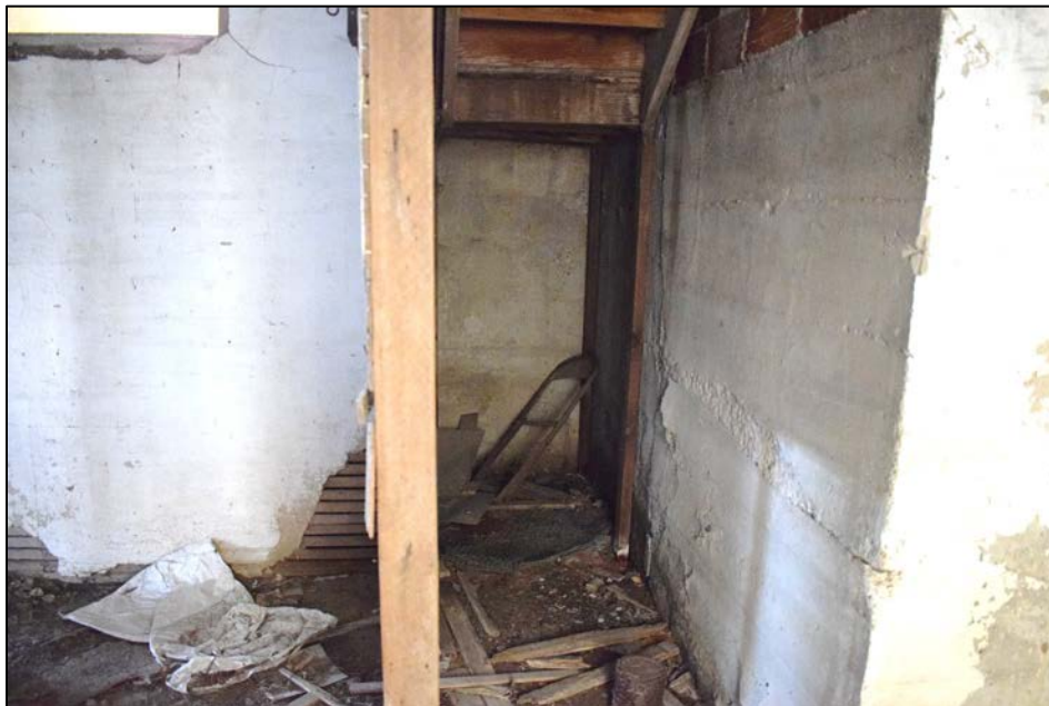
Figure 39. North portion of basement room facing north, opposite boys' toilet.
