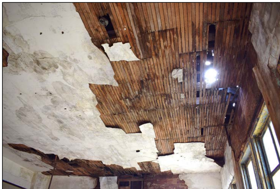
Figure 32. Ceiling details in northwest corner of interior QCRS-MC2A.
