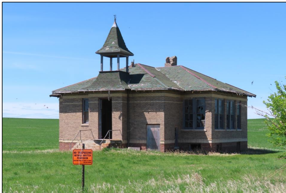
Figure 5. View of front and north sides of QCRS-MC2A facing west-southwest.
