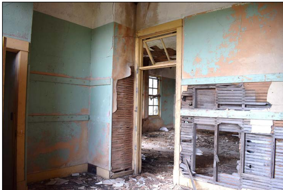
Figure 19. Inside QCRS-MC2A front door in vestibule facing southwest into classroom.
