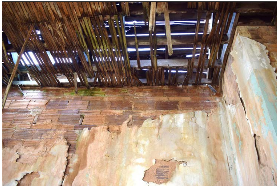
Figure 31. Ceiling details slightly south of center of rear wall in QCRS-MC2A.
