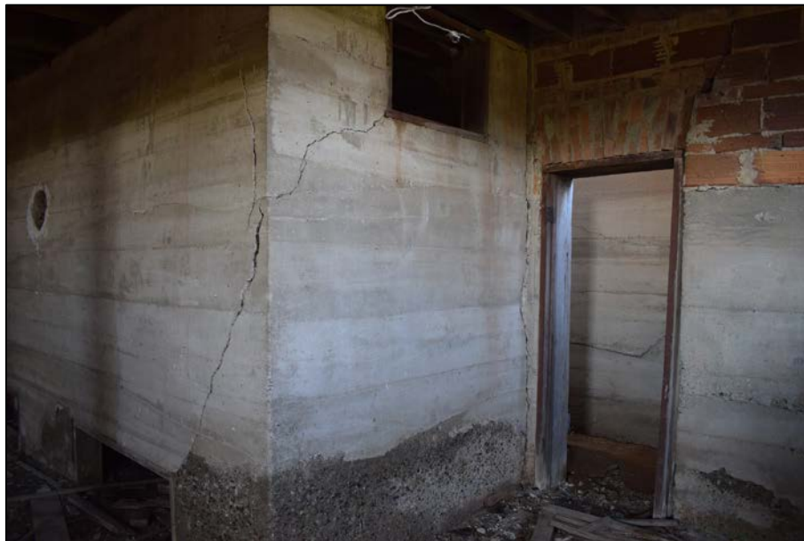
Figure 43. Doorway into rear addition, facing southwest.
