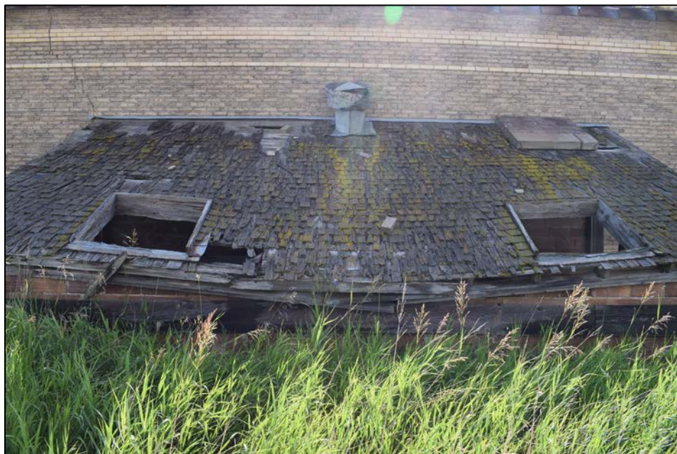
Figure 12. Roof details on addition to rear of QCRS-MC2A facing east
