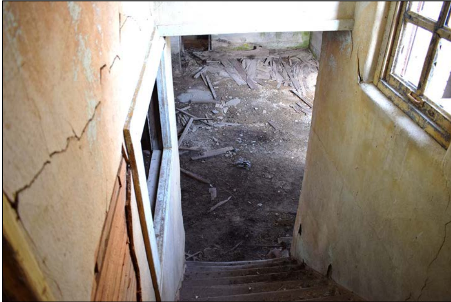
Figure 35. Stairway from vestibule to basement in northeast corner of QCRS-MC2A.
