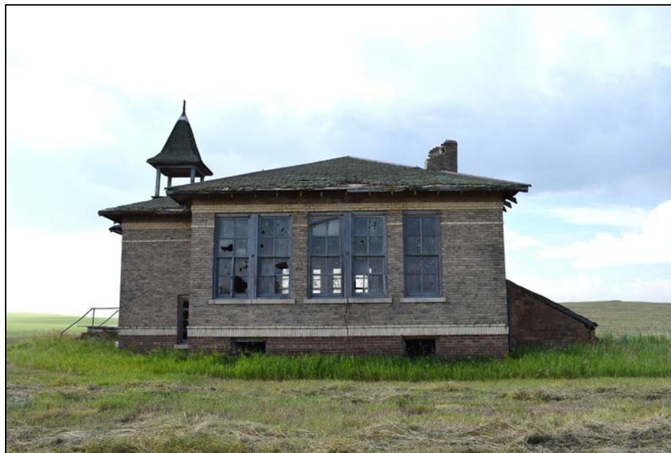
Figure 7. View of north side of QCRS-MC2A facing south.
