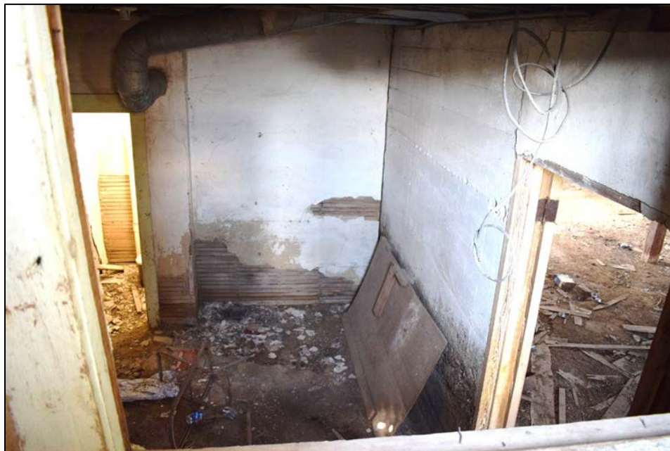
Figure 36. View into basement through interior window in stairwell facing south.
