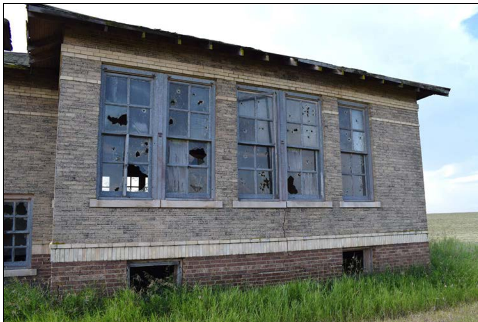
Figure 9. Detail of windows on north side of QCRS-MC2A facing south.
