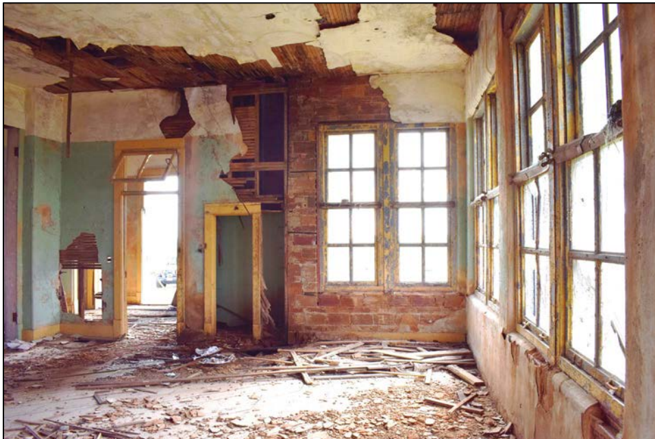
Figure 28. Southwest corner QCRS-MC2A facing east showing window and wall details.
