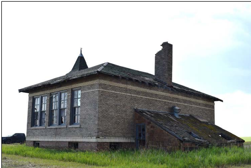
Figure 6. View of rear and north side of QCRS-MC2A facing southeast.
