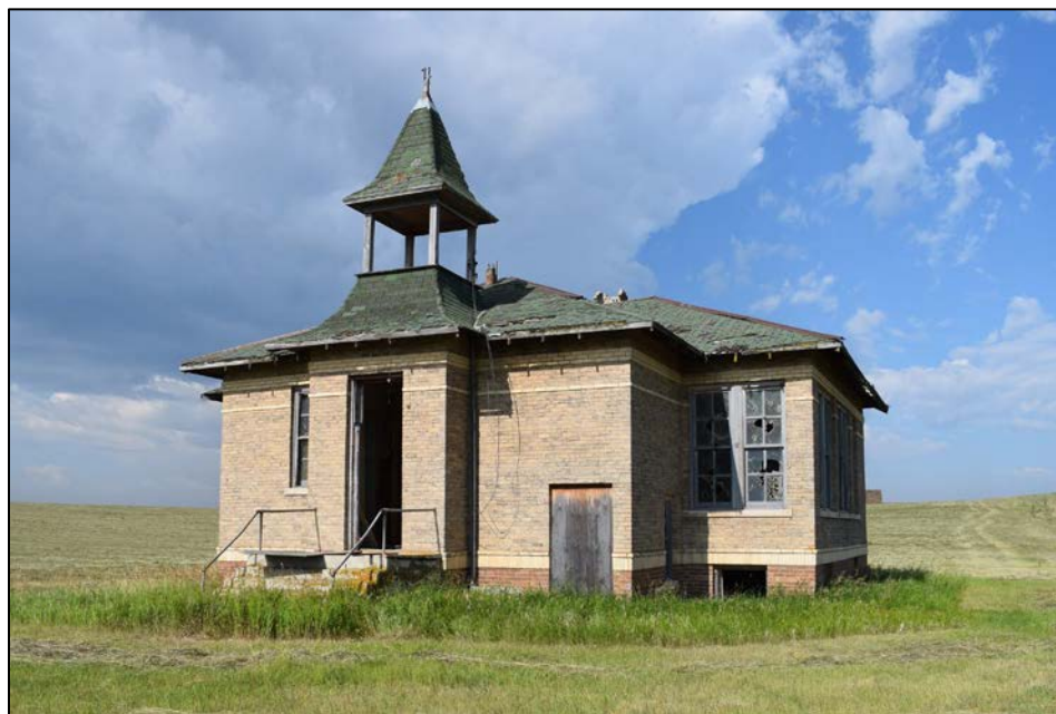
Figure 8. View of front and north side of QCRS-MC2A facing southwest.
