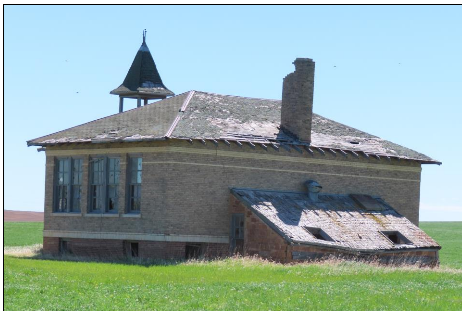
Figure 6. View of rear and north sides of QCRS-MC2A facing east-southeast.
