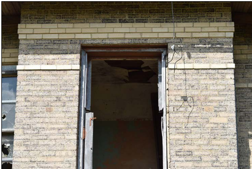
Figure 18. Detail of doorframe on front of QCRS-MC2A facing west.
