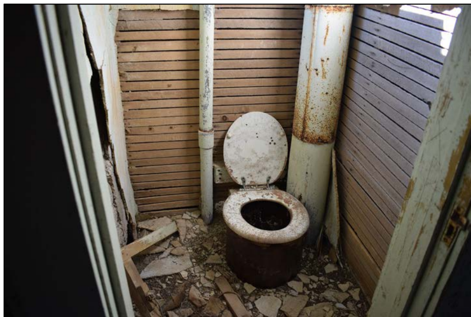
Figure 40. Boys' toilet in basement facing south.
