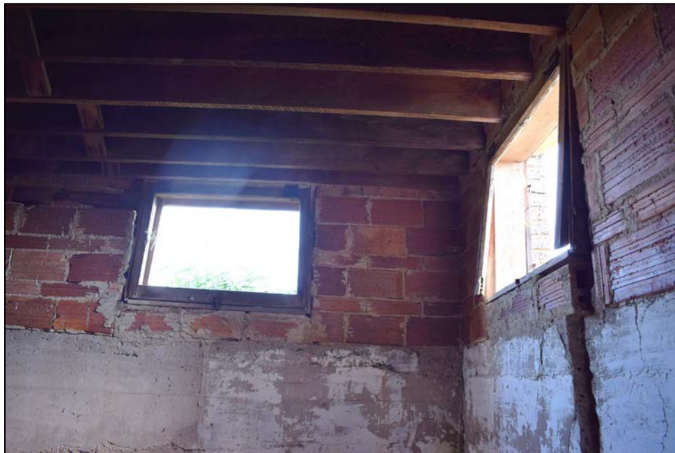
Figure 48. Northeast basement windows facing north.
