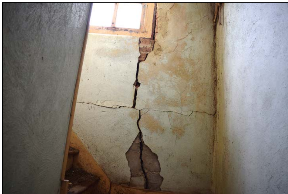
Figure 24. Facing east up stairway from girls' toilet in QCRS-MC2A.
