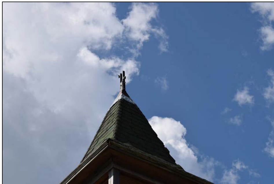
Figure 16. Detail of flagpole attachment on bell tower of QCRS-MC2A facing southeast.
