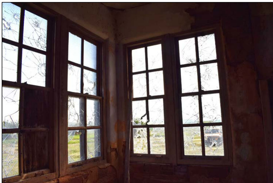
Figure 30. North and east window details facing northeast in QCRS-MC2A.
