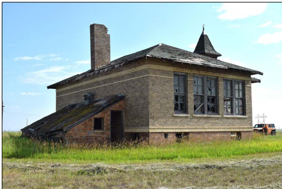
Figure 4. View of rear and south side of QCRS-MC2A facing northeast.
