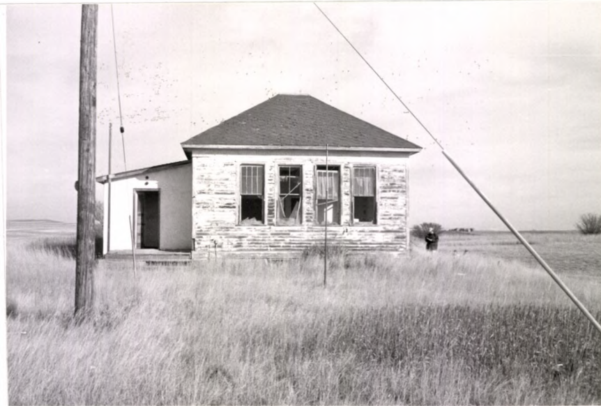
View to north Kid Creek School (roll #10/14/96, exposure #8).
