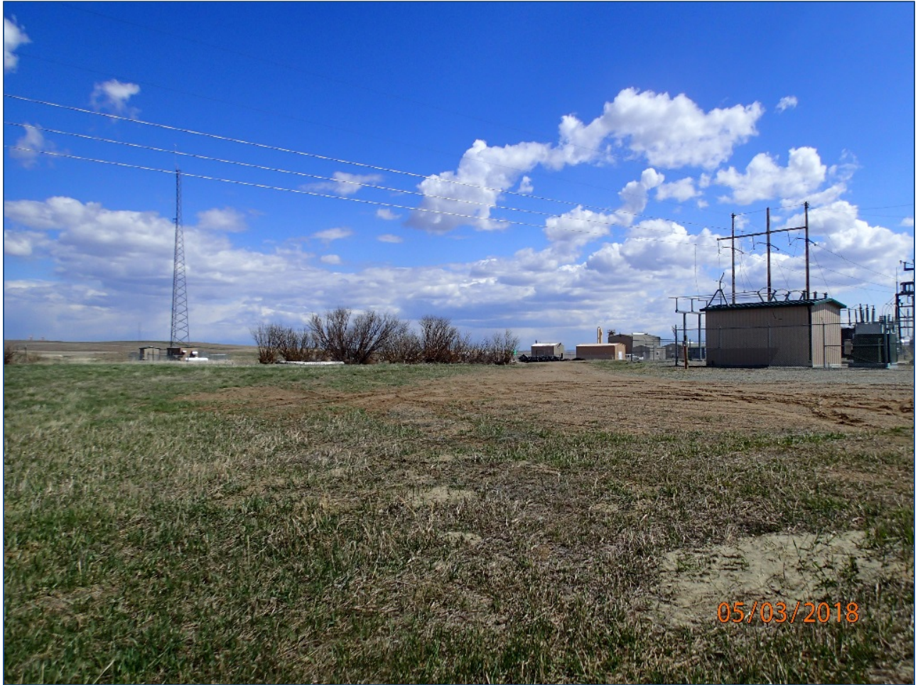
Figure 1: Former location of site 32BO962. View to the southeast. Area is currently an electrical substation.
