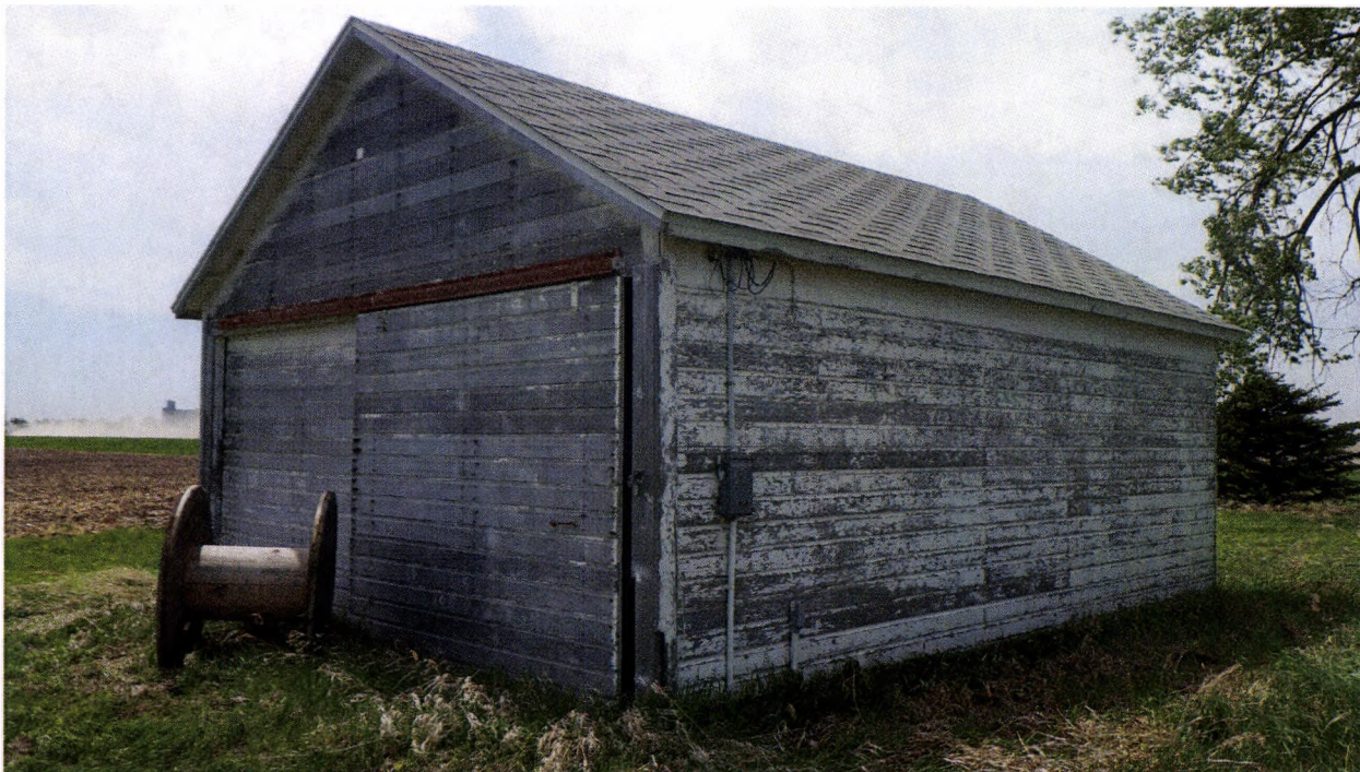
Figure 1: View to the southwest over MAC-NB-4x (Image 2815).
