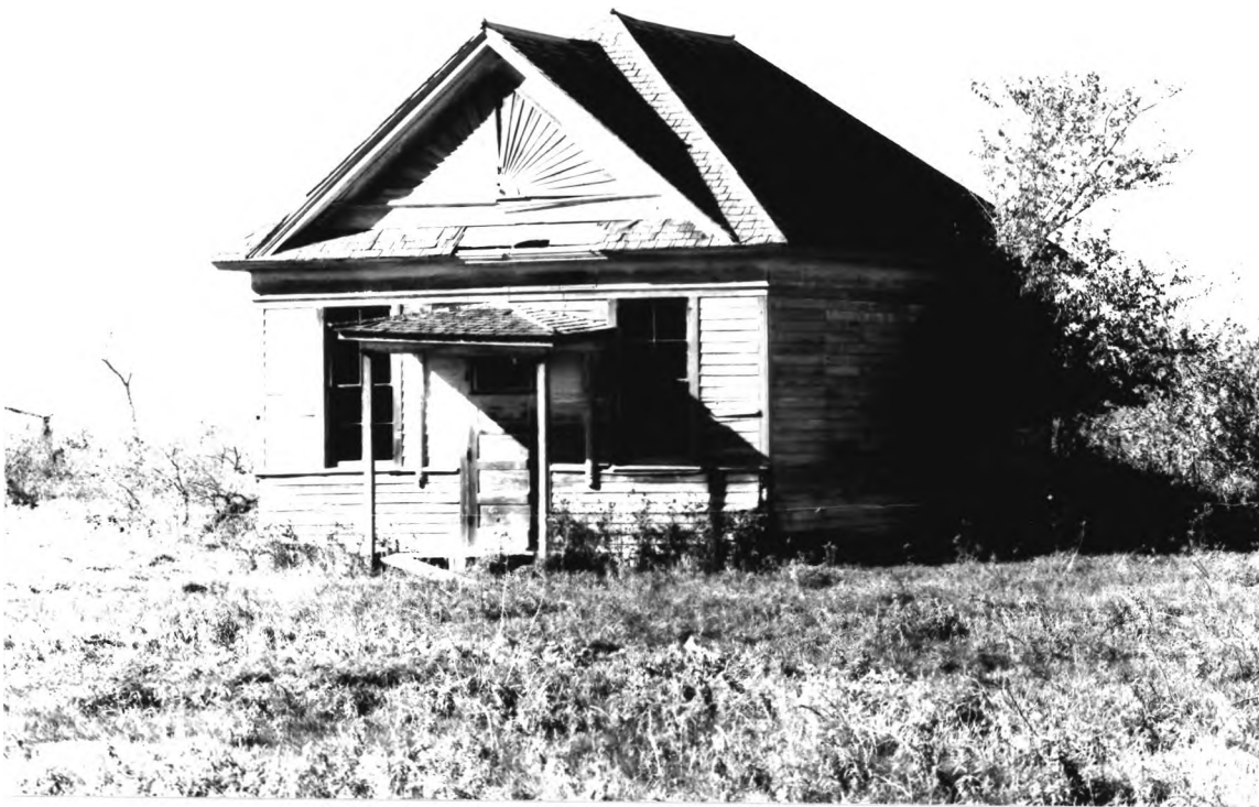
Photograph #2: Schoolhouse Looking West (Roll 1, Neg. 20)
