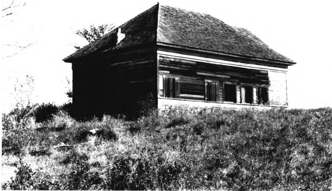
Photograph #4: Schoolhouse Looking Northeast (Roll 1, Neg. 22)
