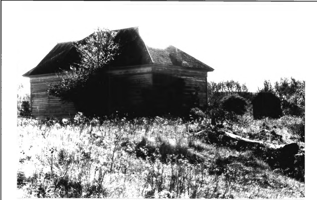
Photograph #5: Schoolhouse Looking Southeast (Roll 1, Neg. 23)
