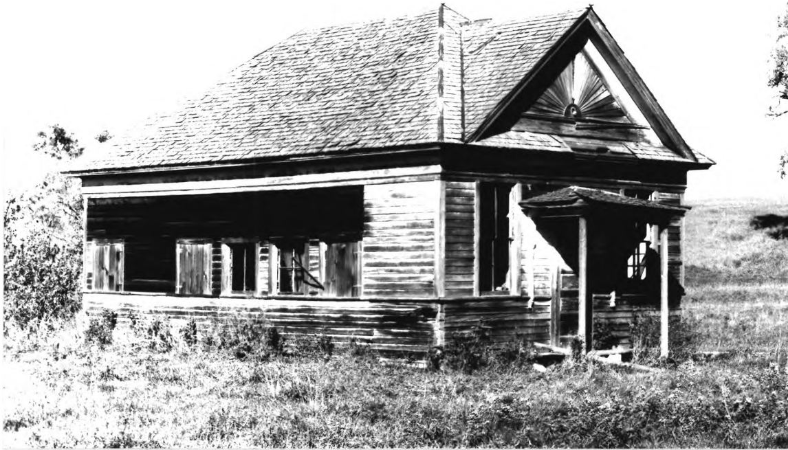
Photograph #3: Schoolhouse Looking Northwest (Roll 1, Neg. 21)
