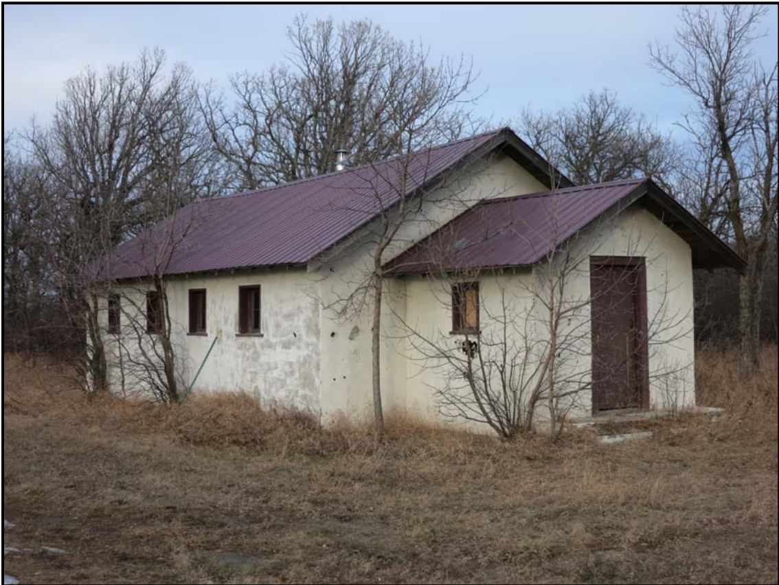
Figure 4: Overview of the southwestern corner of Feature 1, view to the northeast.
