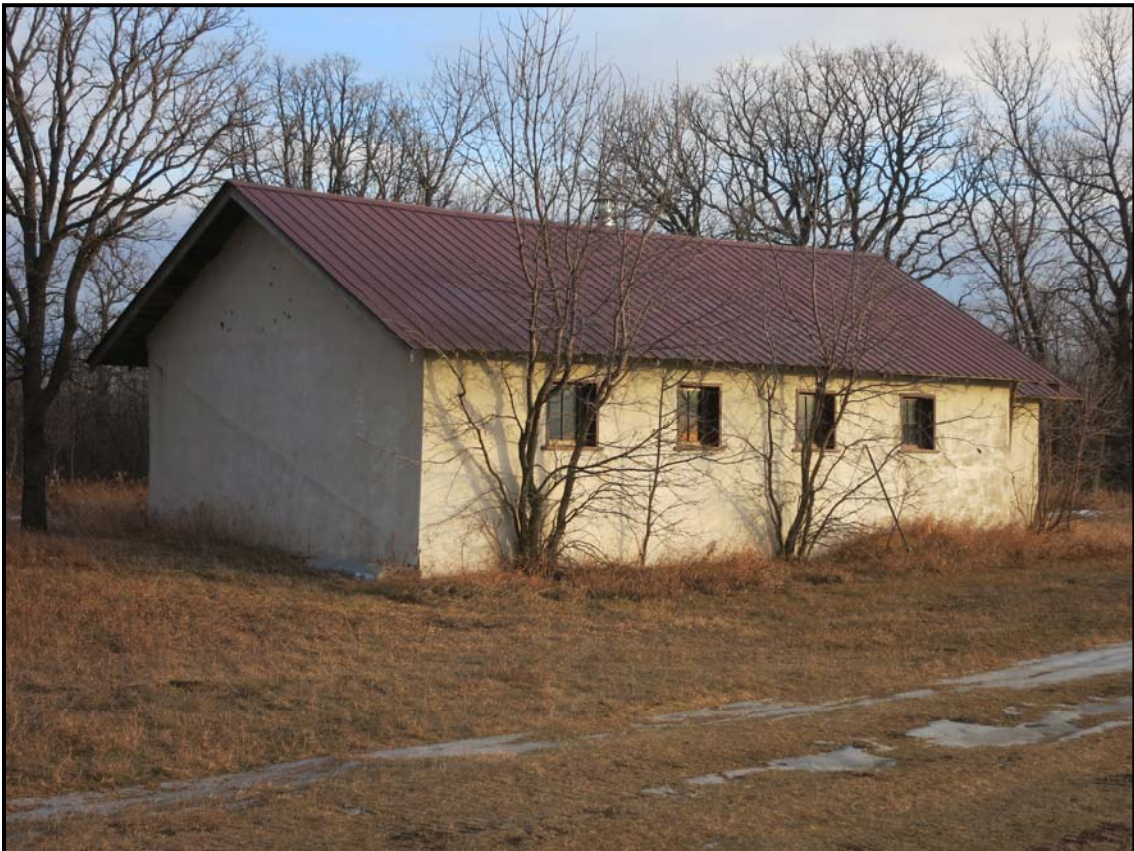
Figure 5: Overview of the northwestern corner of Feature 1, view to the southeast.
