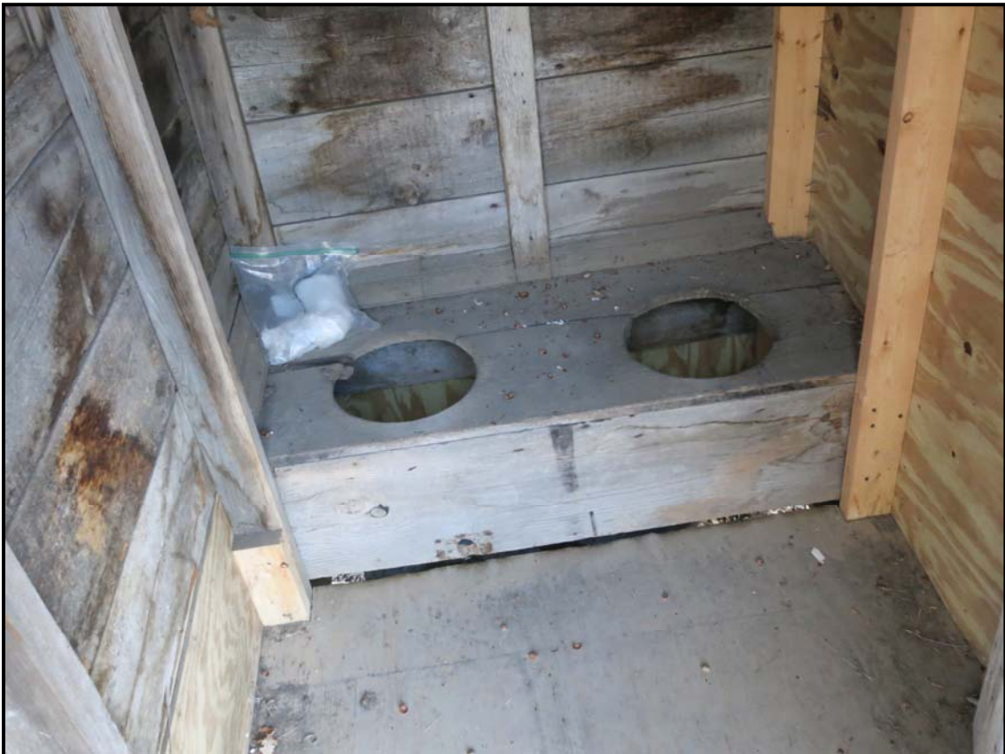
Figure 9: Overview of the interior of Feature 3. Note the modern repairs to the structure.
