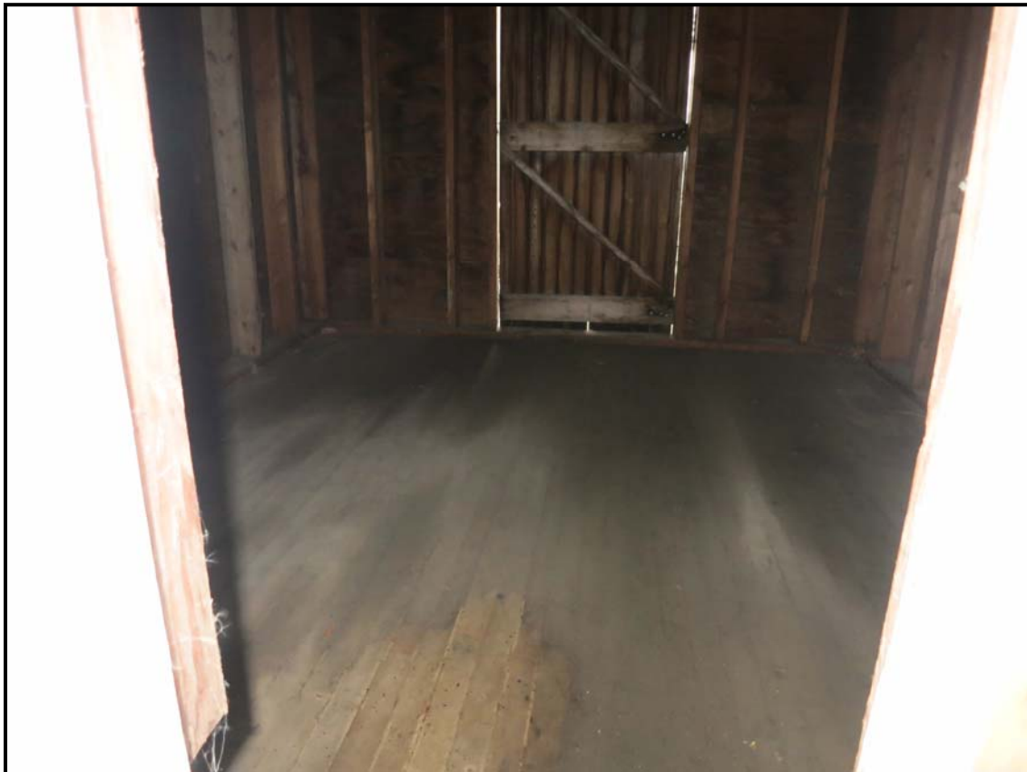
Figure 7: Overview of the interior of Feature 2, facing west.
