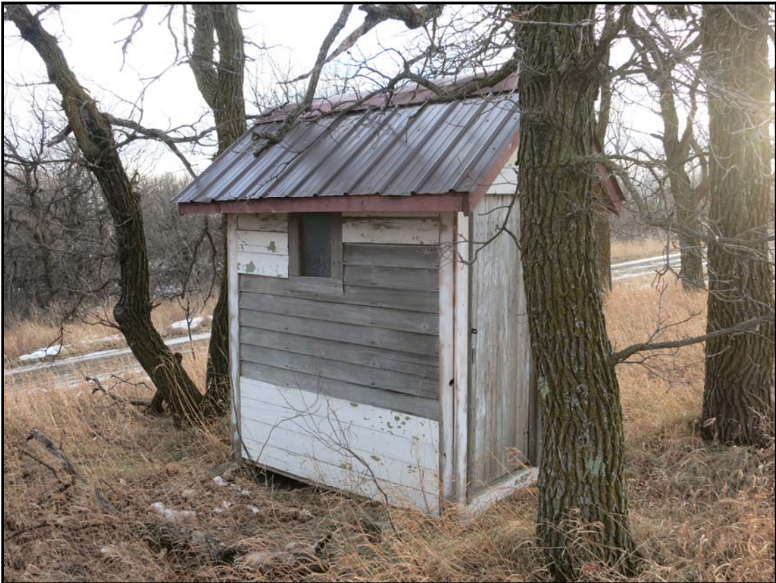
Figure 8: Overview of Feature 3 at Site JUP-17090-303, view to the southwest.
