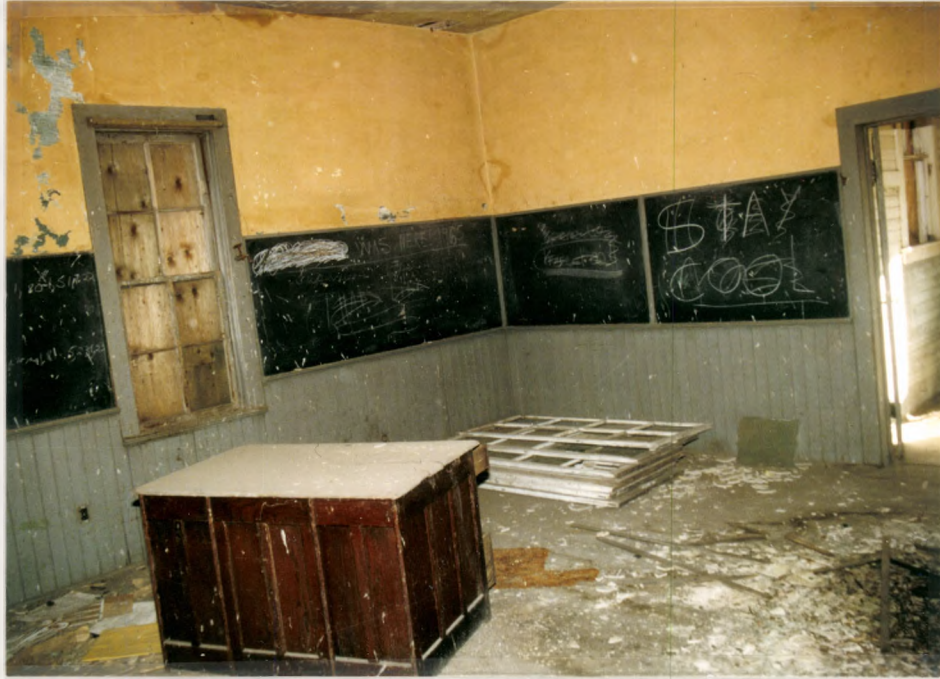
9. VIEW FR. FRONT ROOM TOWARDS ENTRY
