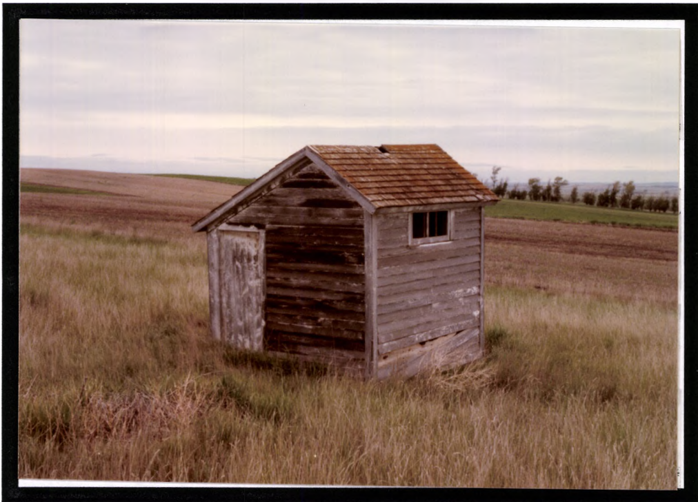
Ridgeway Community Center one of the outhouses
