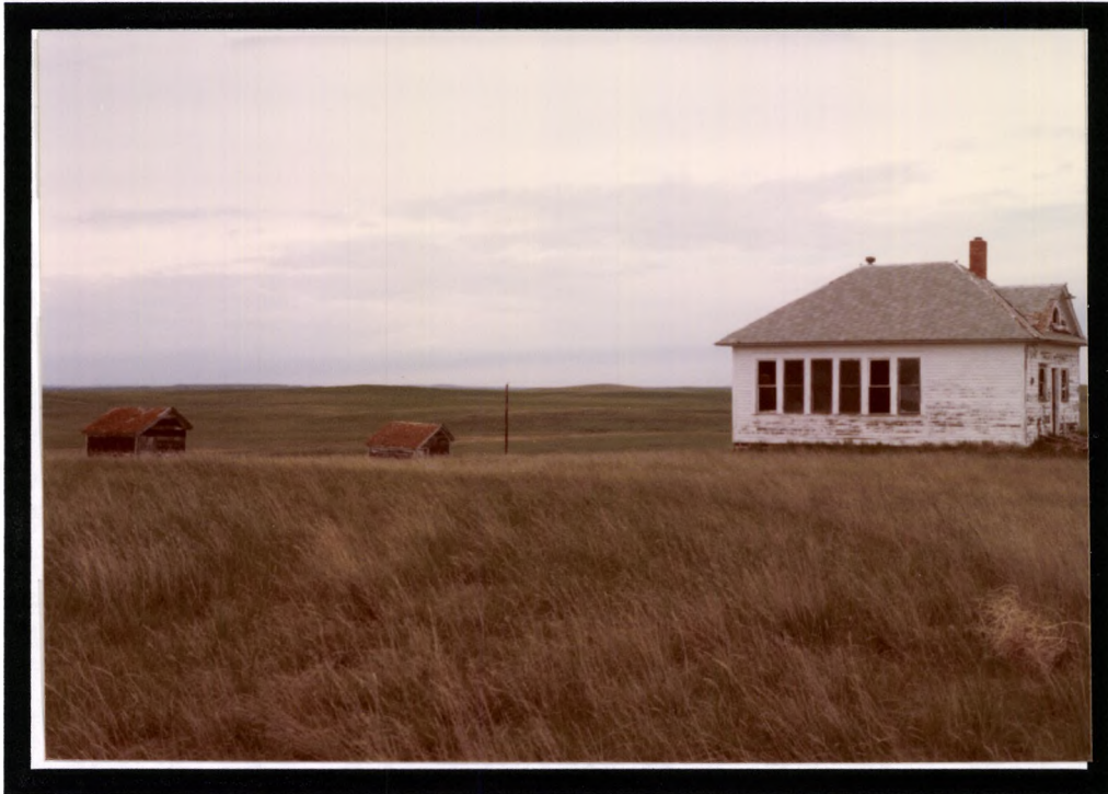
Ridgeway Community Center overview from southeast note location of outhouses
