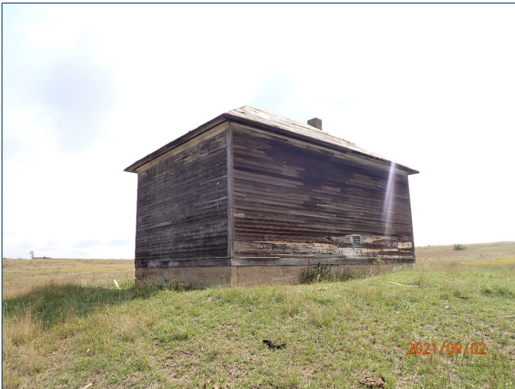
Figure 5. West and north elevation of the schoolhouse, looking southeast.
