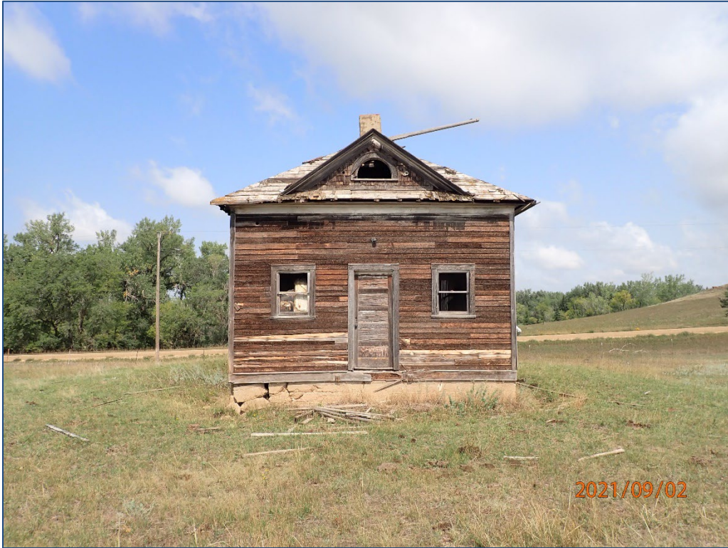
Figure 2. Front (south) elevation of the schoolhouse, looking north.
