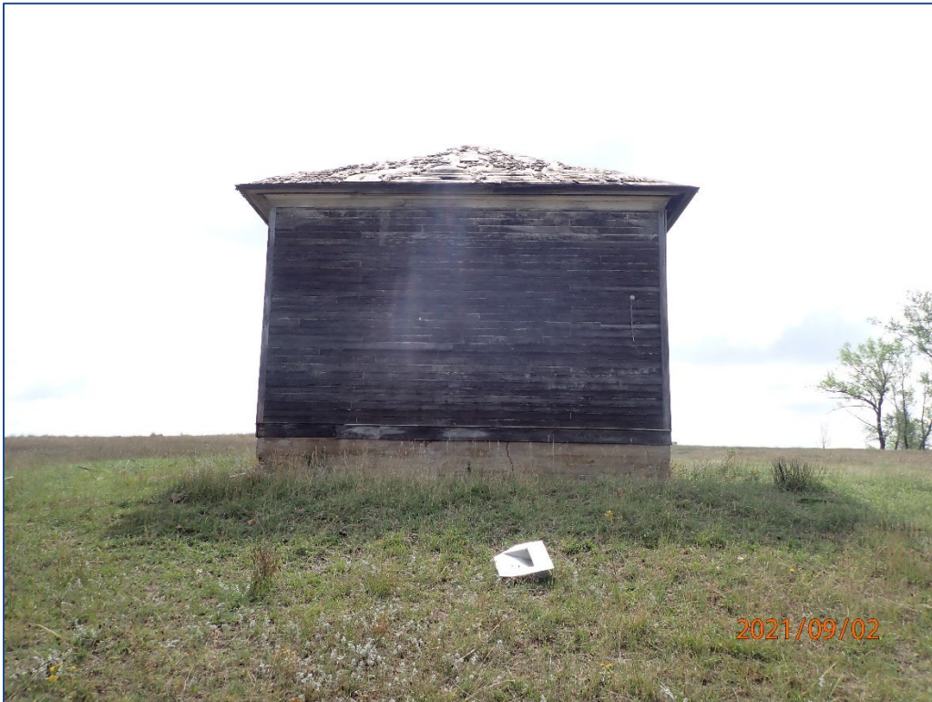
Figure 6. Rear (north) elevation of the schoolhouse, looking south.
