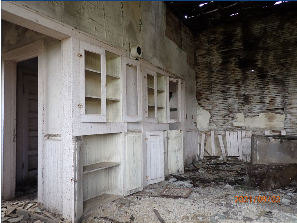
Figure 10. Interior view of the schoolhouse, looking southwest.
