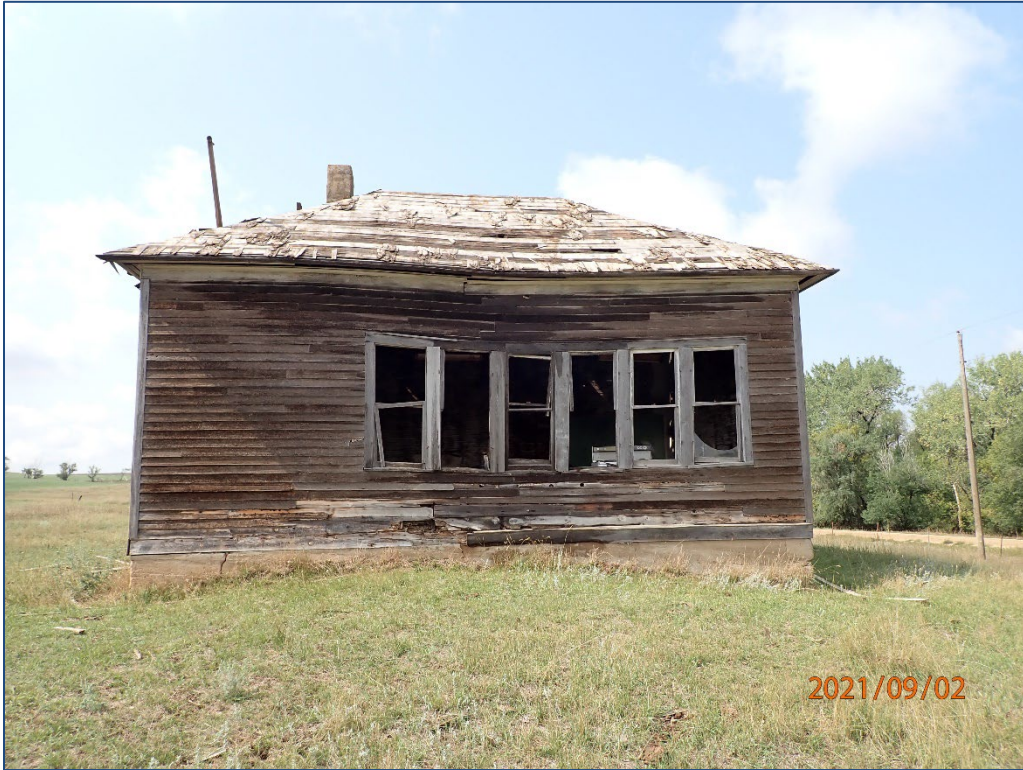
Figure 8. East elevation of the schoolhouse, looking west.
