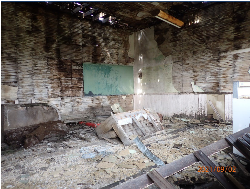
Figure 11. Interior view of the schoolhouse, looking northwest.
