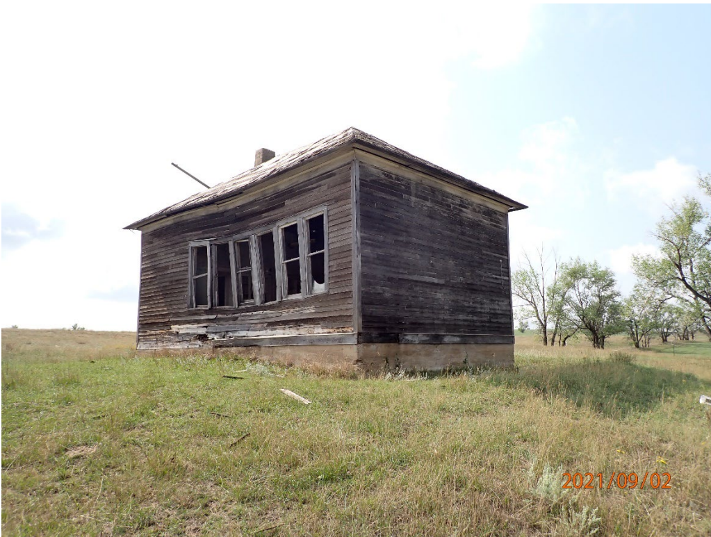
Figure 7. East and north elevation of the schoolhouse, looking southwest.
