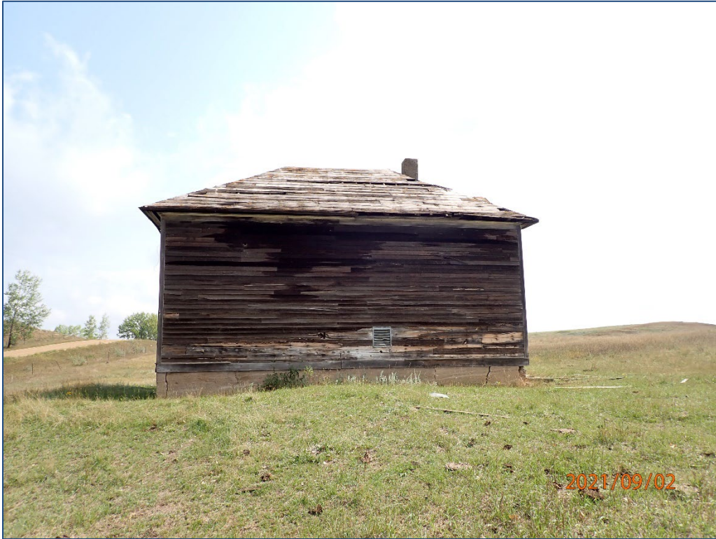
Figure 4. West elevation of the schoolhouse, looking east.
