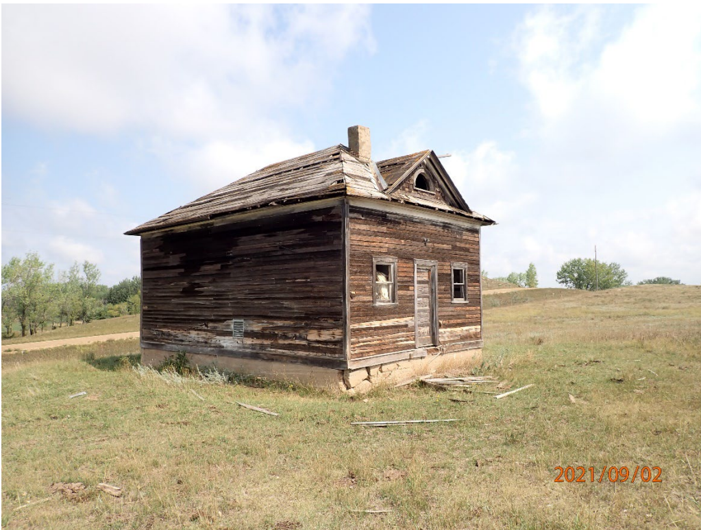
Figure 3. South and west elevation of the schoolhouse, looking northeast.
