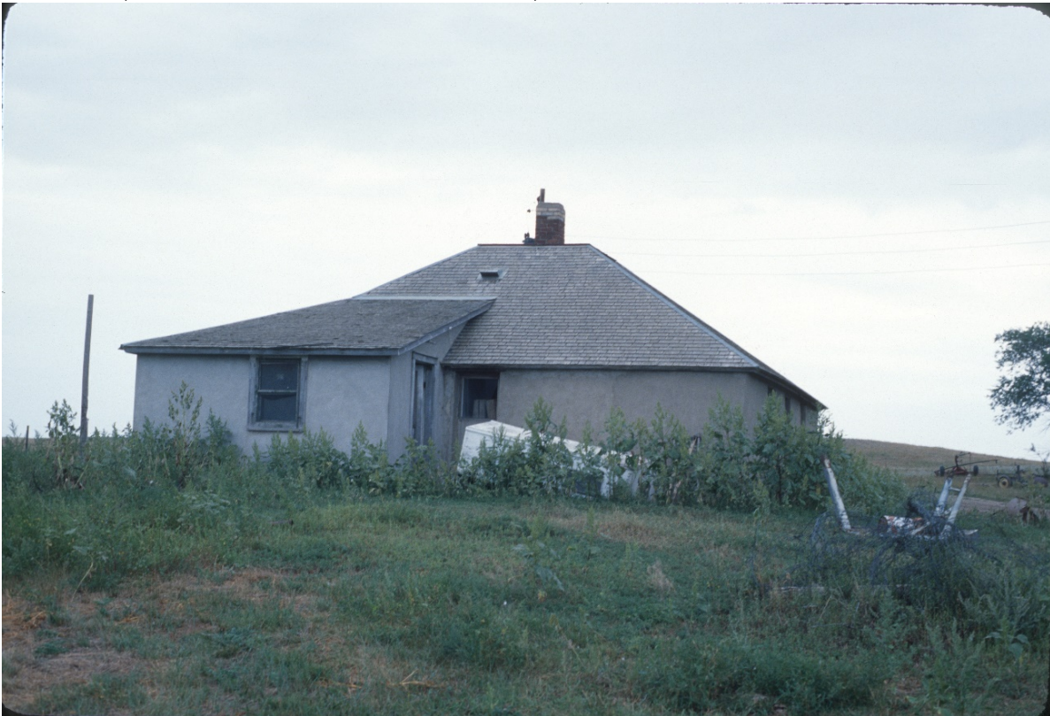
Feature 1 from south, scanned from AHP Photo Collection, taken 1979
