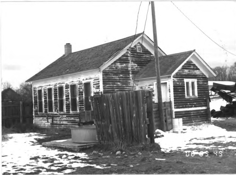
Feature 19 - View To The Southeast
