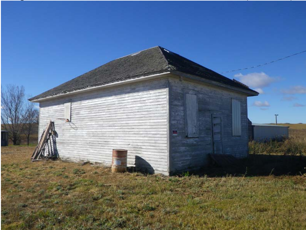
Figure 3: Site lead MAC-KEM-x01, Feature 1, view southwest (IMPG0578).
