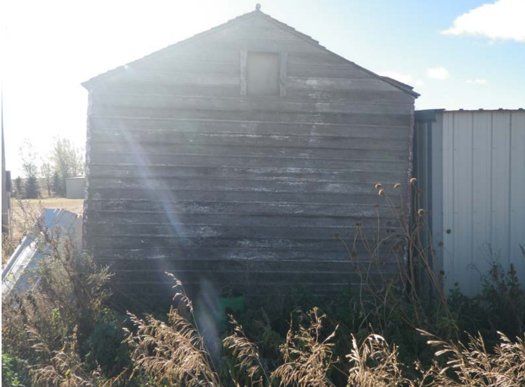
Figure 5: Site lead MAC-KEM-x01, Feature 2, view south (IMPG0584).
