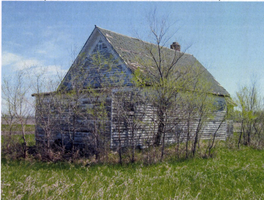
May 18, 2011 view to southeast of north and west elevations.
