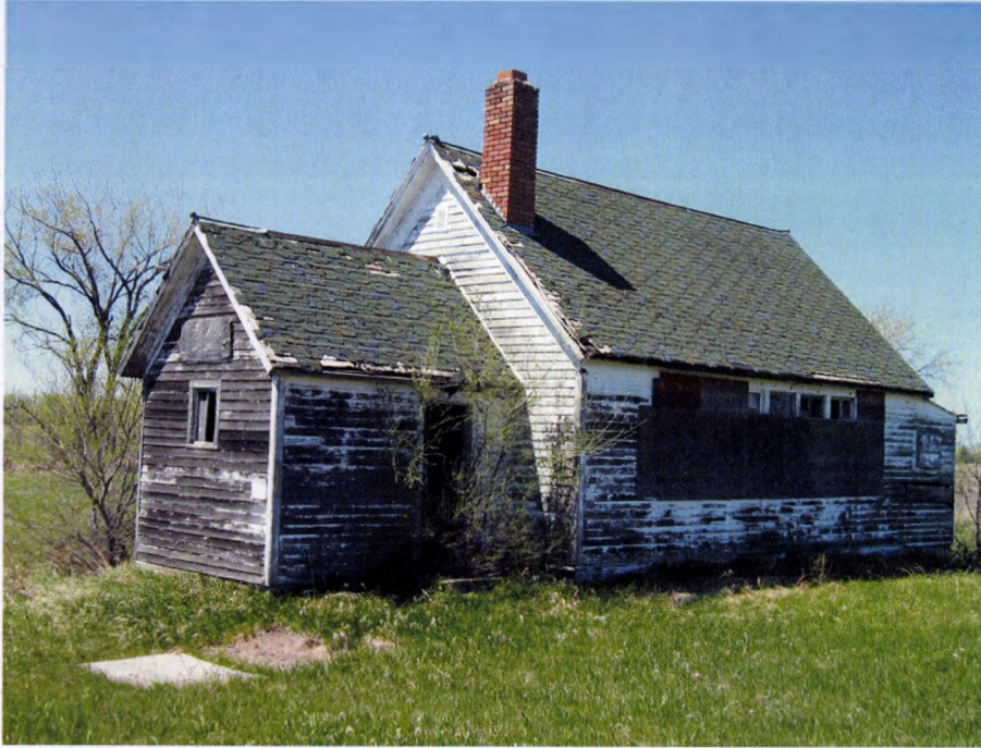
May 18, 2011 view to northwest of south elevation and east façade.
