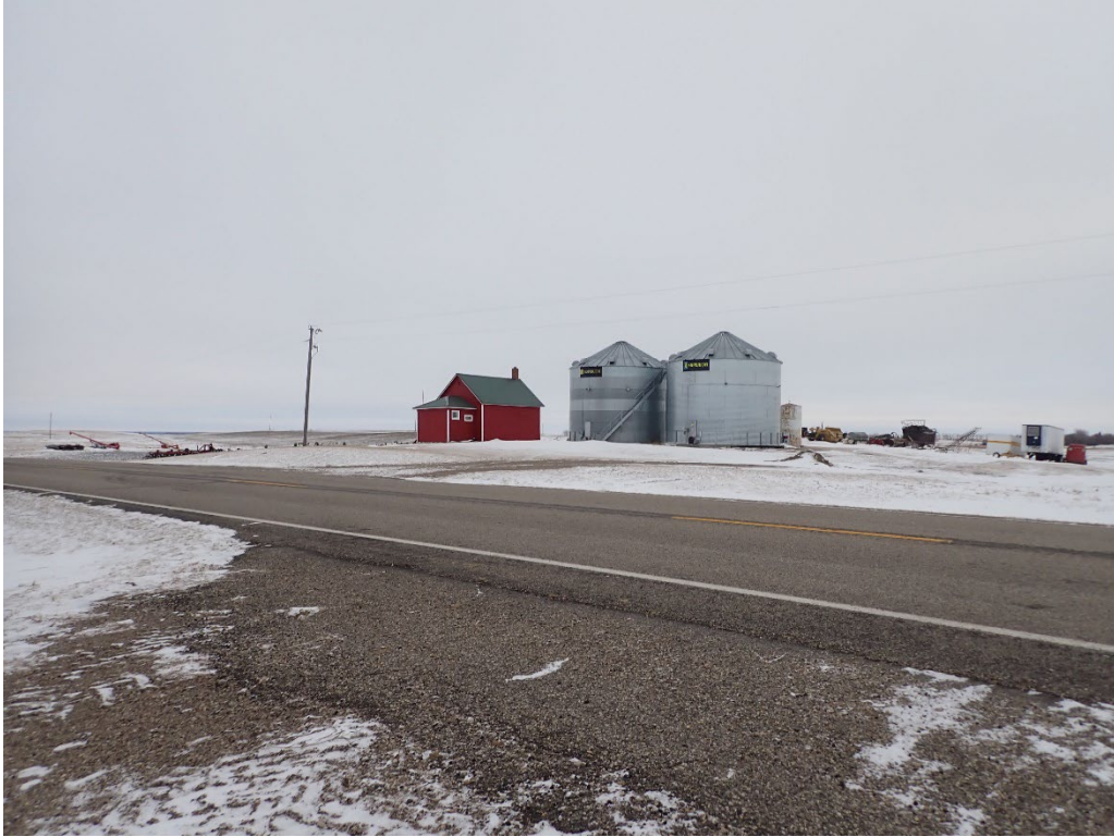
Figure 3: Feature 1, view to the southeast.
