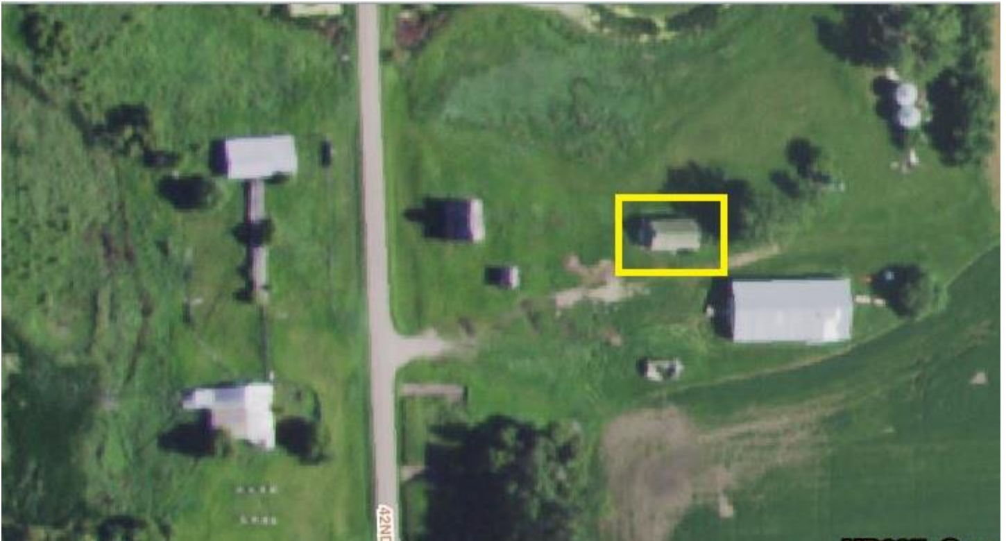
Figure 1: 2020 aerial imagery of 32GF3818
