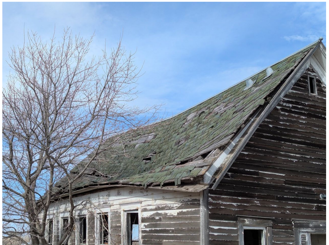
Roof on the West Side
