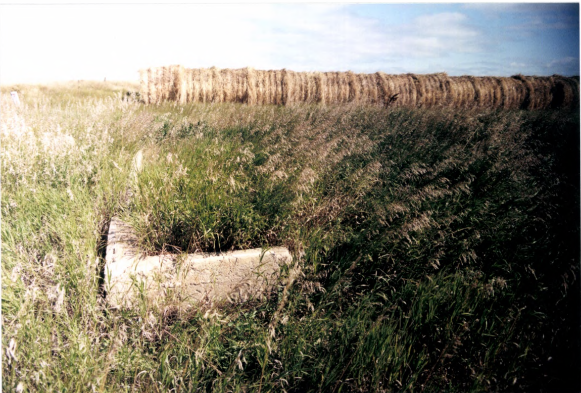
Concrete foundation, view north (SWPL05-CP176).
