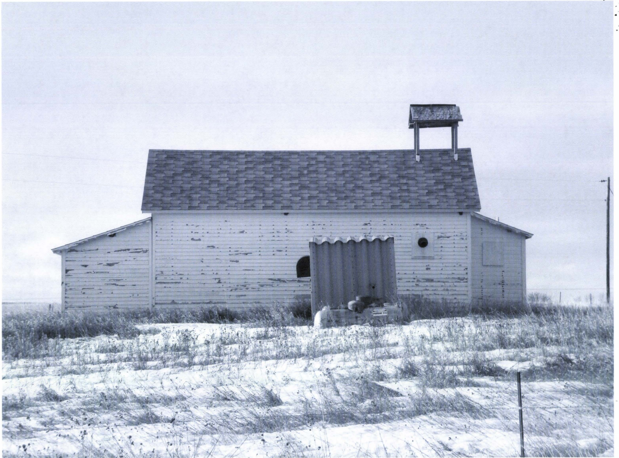
Haynes Township School North 3/22/2010 North Side Kathy Wilner KD
