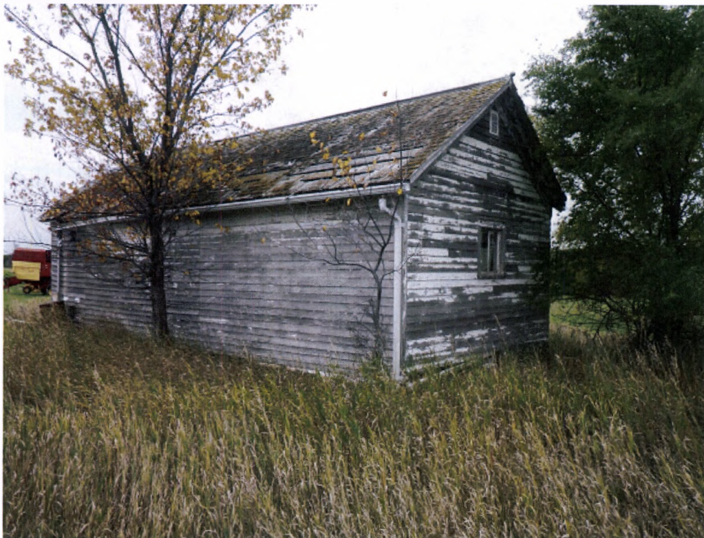
Figure 3: Overview of feature 1 (northeast corner), view to the southwest.
