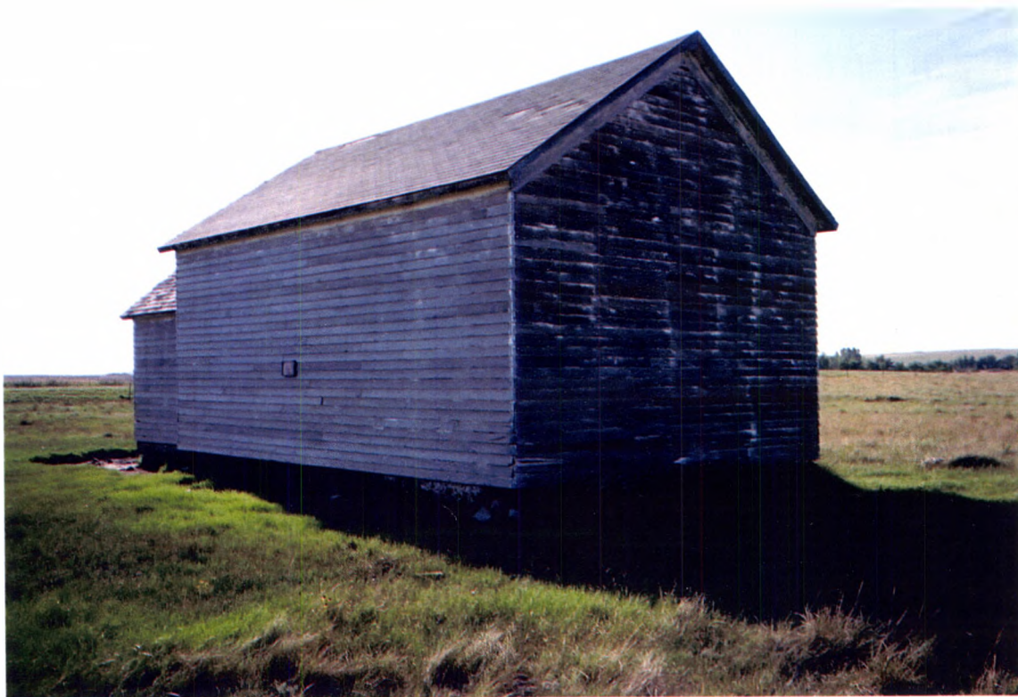
Feature 1, view to the southeast
