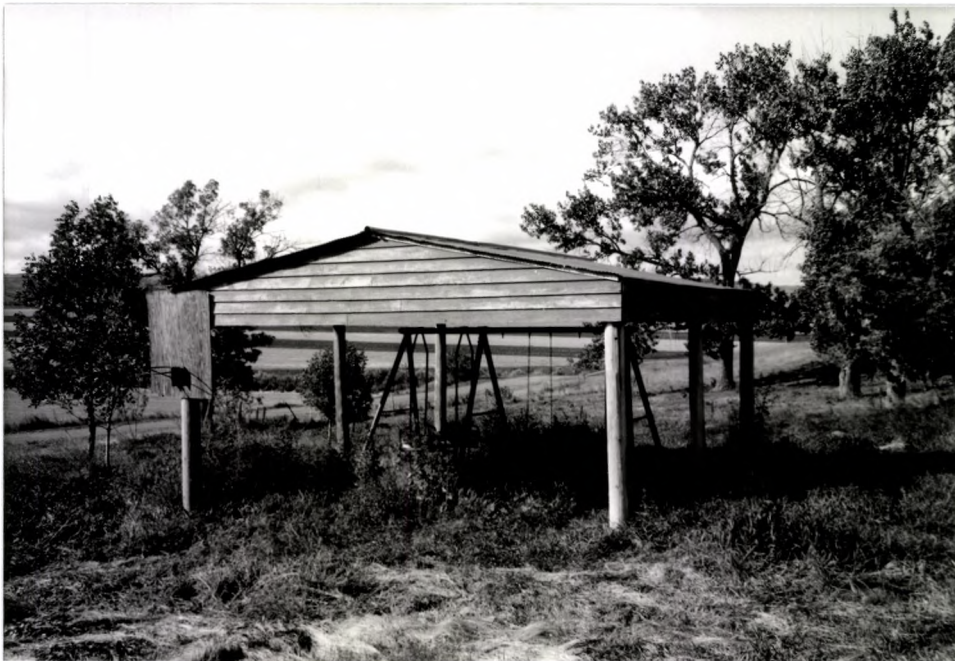
FEATURE 3: Shelter, view to southwest
