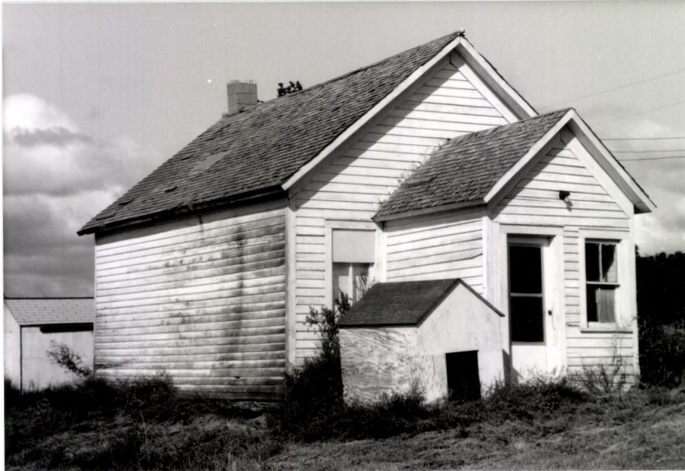
FEATURE 2: Schoolhouse, south and east elevations, view to west
