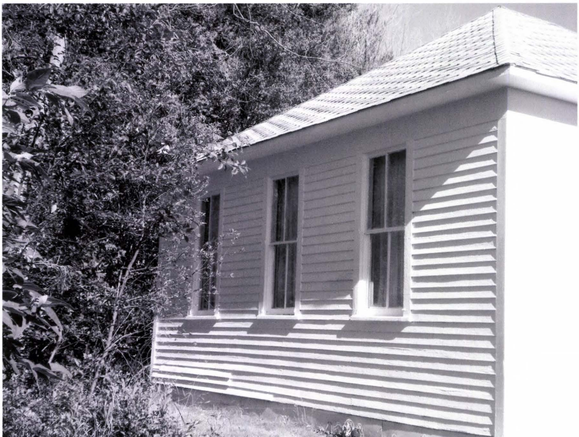
Villard School #4 South Side 06/14/2012 Kathy Wilner MH
