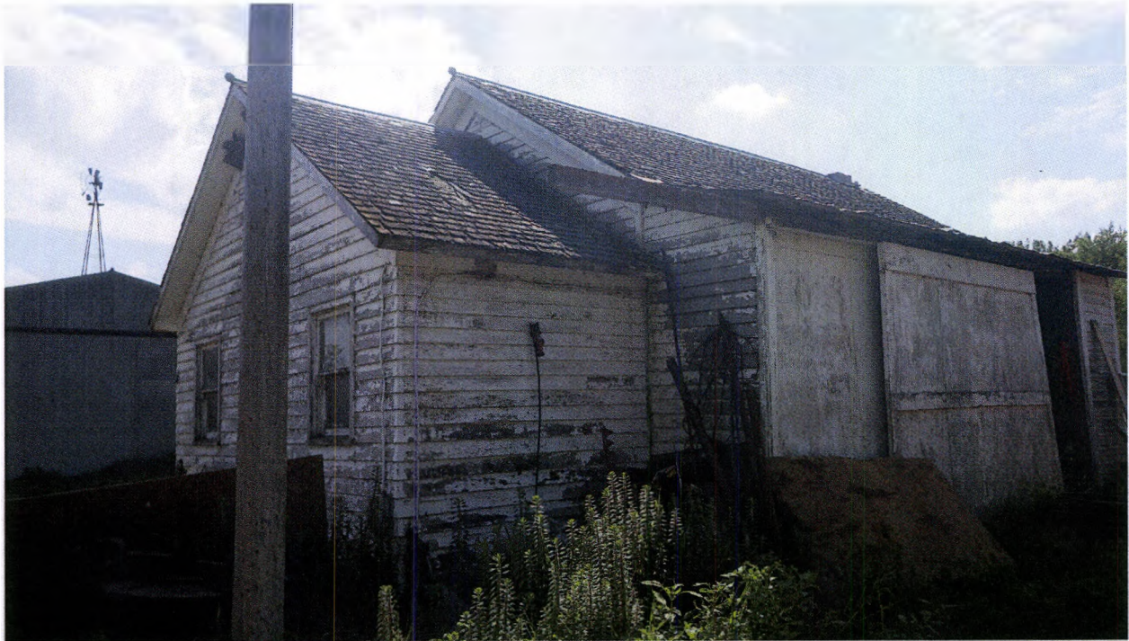
Figure 8: View of MAC-UP-43x, to the northeast, Feature 3 (Image 0915).
