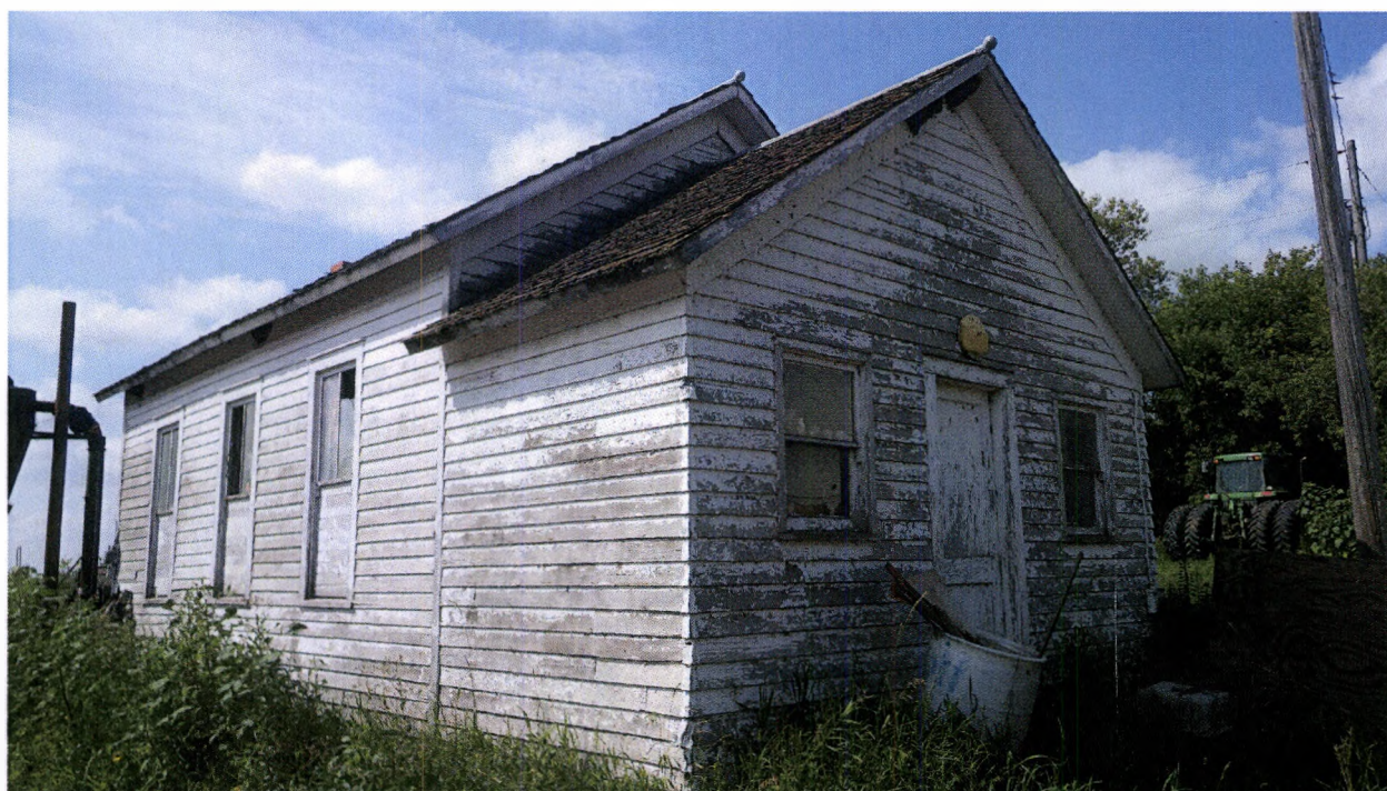
Figure 7: View of MAC-UP-43x, to the southwest, Feature 3 (Image 0909).
