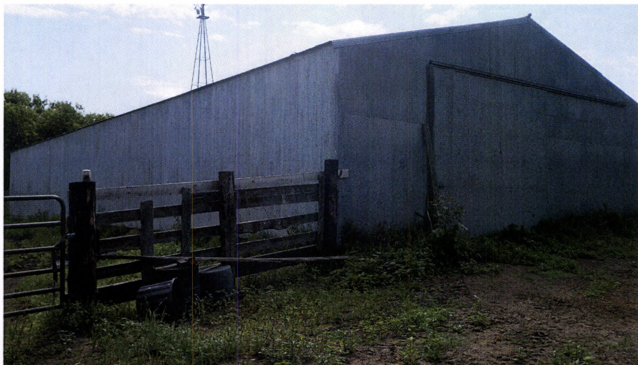
Figure 6: View of MAC-UP-43x, to the southeast, Feature 2 (Image 0892).
