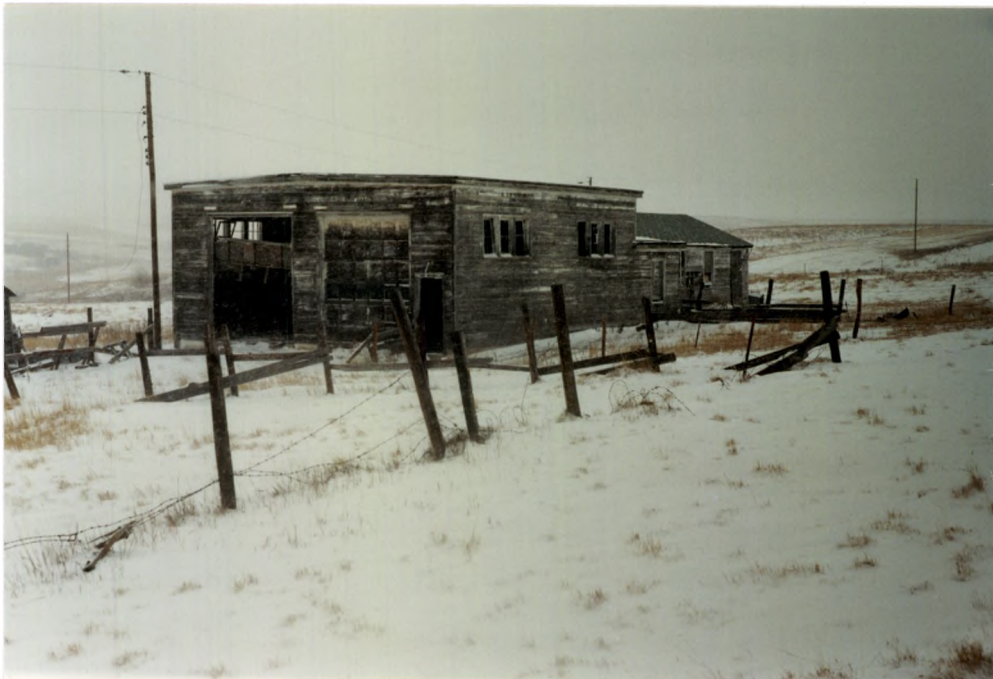
Feature 1, south and east elevations, view to the northwest; 970919c, Roll 100, Negative 20.
