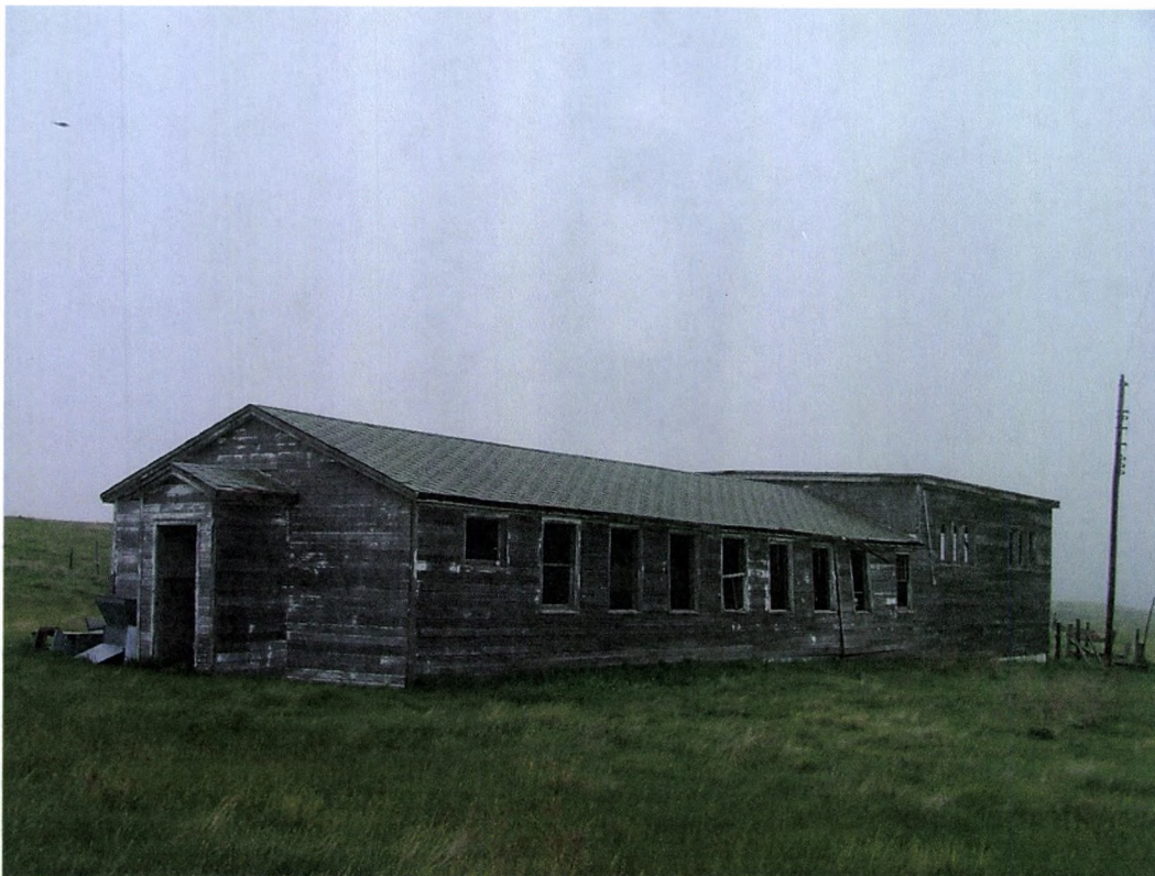
Feature 1, view to the southeast
