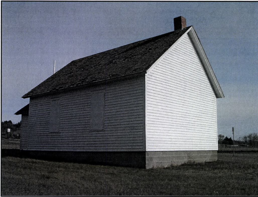
Figure 9: Overview of the southwestern corner of the Nettle Creek School, view to the northeast.
