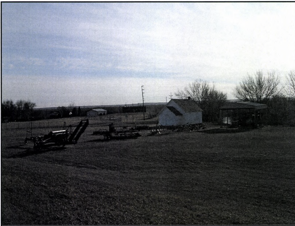
Figure 3: Overview of Nettle Creek School and associated features, from northwest of the school, view to the south-southeast.
