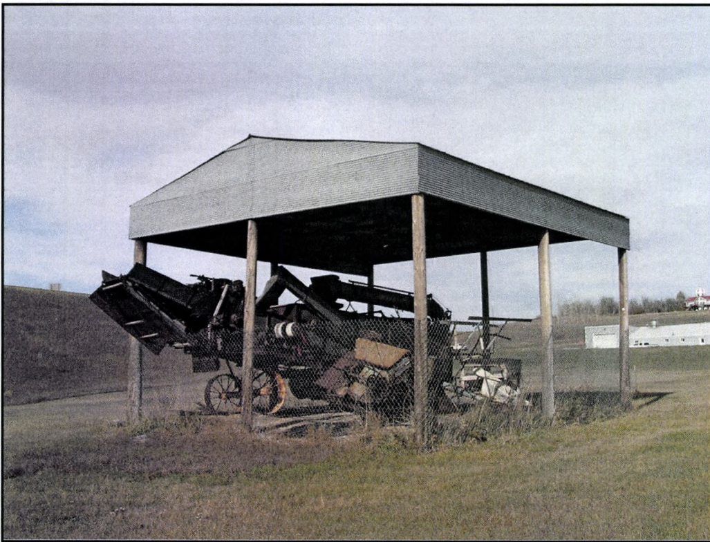
Figure 12: Overview of the southeastern corner of the machinery shed, view to the northwest.
