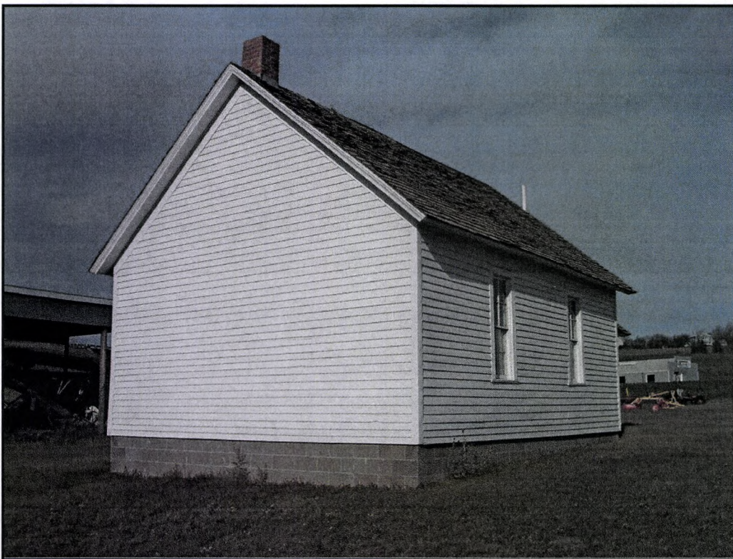
Figure 8: Overview of the southeastern corner of the Nettle Creek School, view to the northwest.
