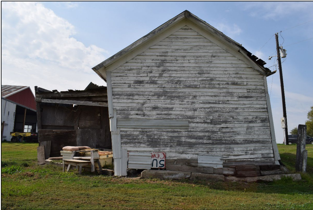
Figure 4. Feature 1 facing west. K. Ward 09/20/2023.
