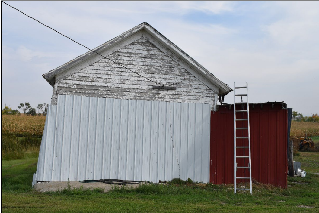
Figure 2. Feature 1 facing east. K. Ward 09/20/2023.
