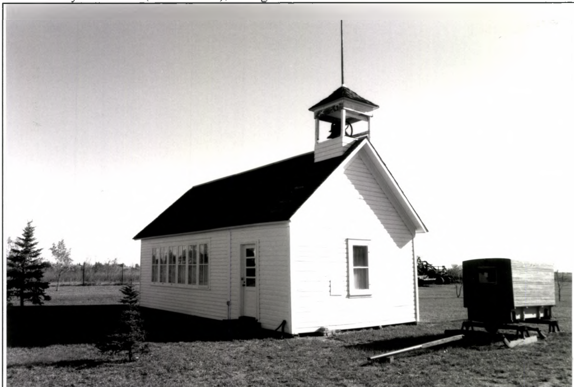
Front of Country School #3 (Feature #13), facing NE
