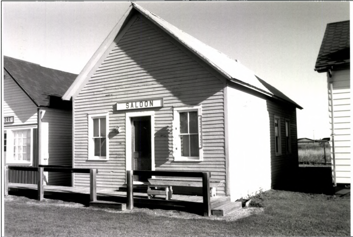
Front of Country School #2 ( Saloon ) (Feature #7), facing NW
