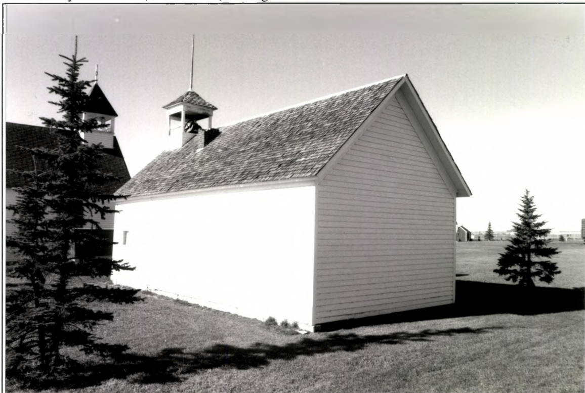
Rear of Country School #3 (Feature #13), facing SW
