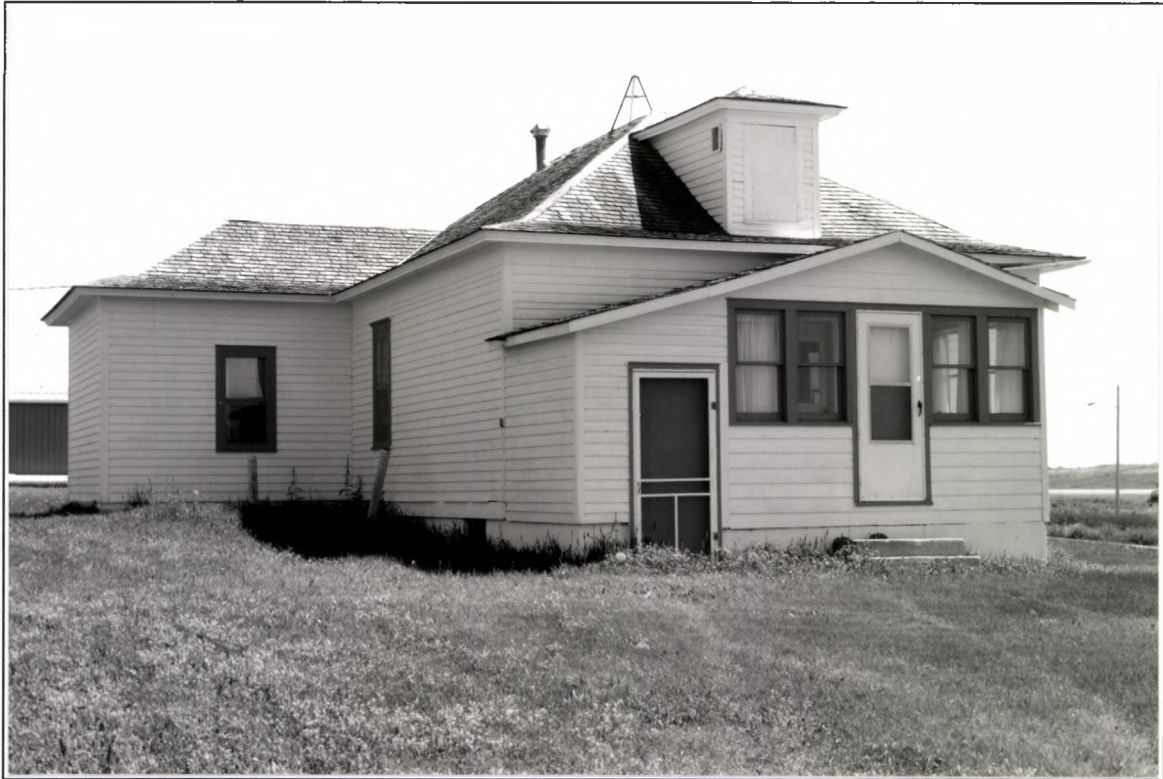
Old Schoolhouse, facing SE
