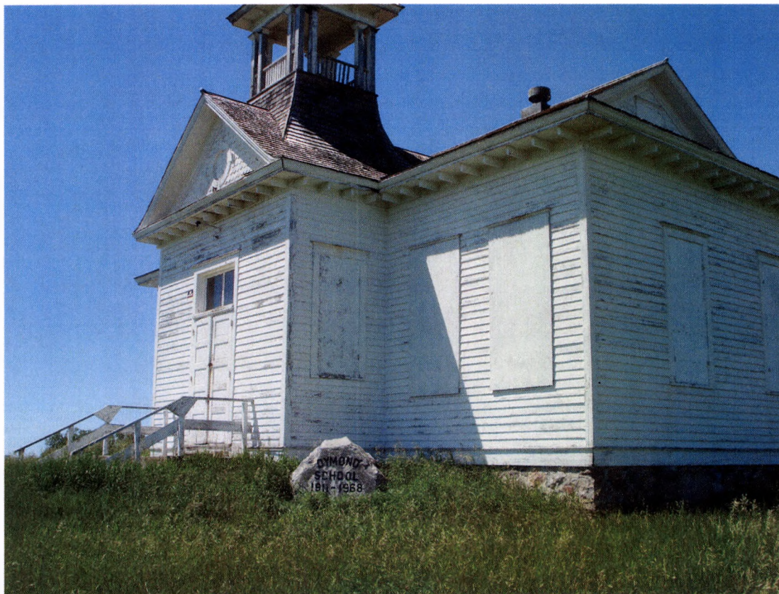
Dymond School, Feature 1, view southwest (#31).
