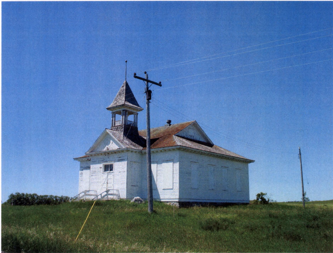
Dymond School, Feature 1, view southwest (#27).
