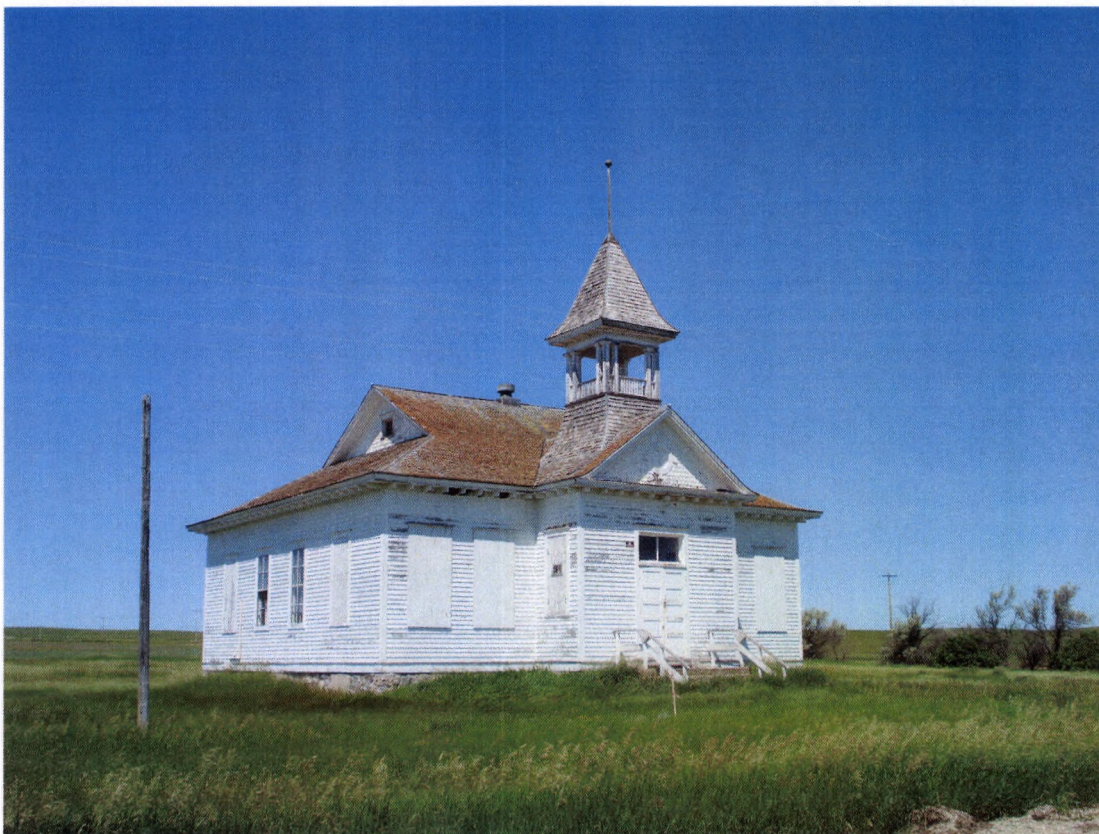
Dymond School, Feature 1, view north northwest (#33).
