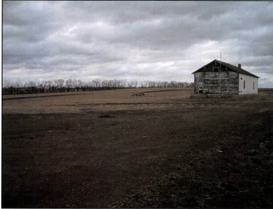
Figure 1. S-SL-1-Fertile LCS site overview, facing northwest.
