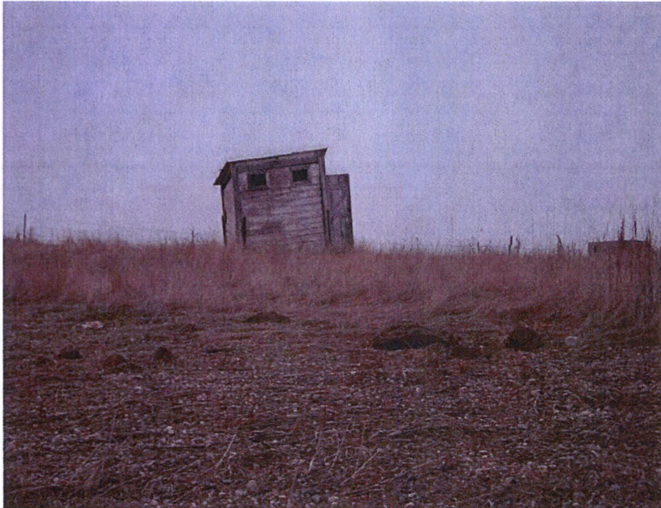
Figure 3: View of MAC-H8-HS2; Feature 2 looking east (Photo #348).
