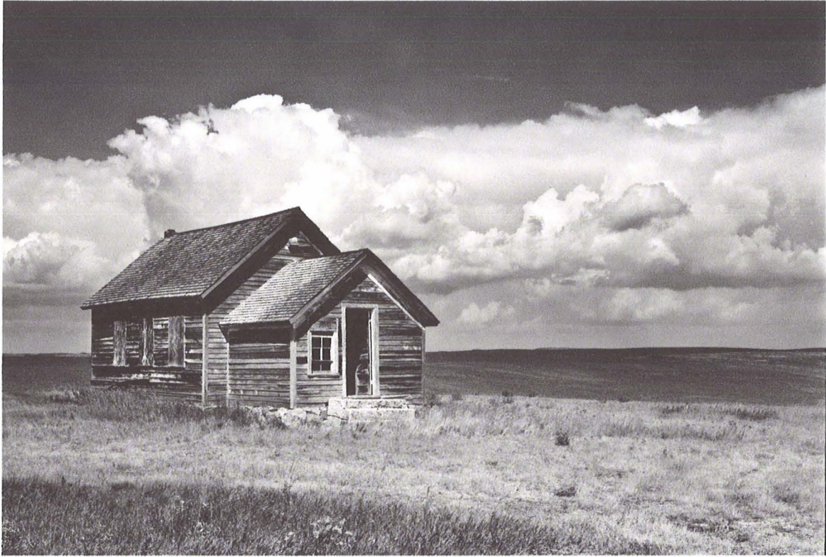
West and South Side
