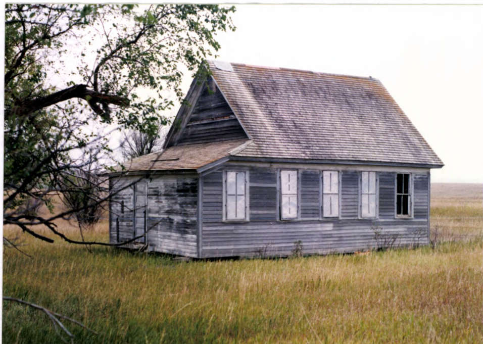
School house, south and west elevations, 960918a Roll 1, Negative 5
