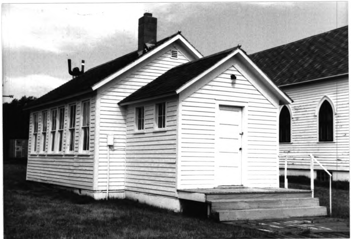
Camera Facing West
