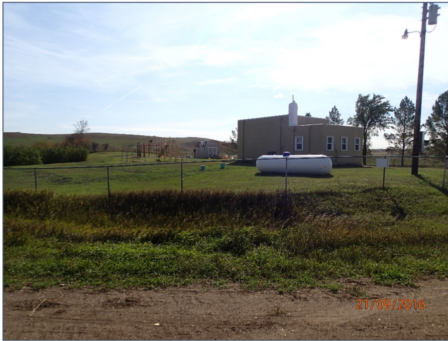
Figure 1. Overview of site. View to the southeast.
