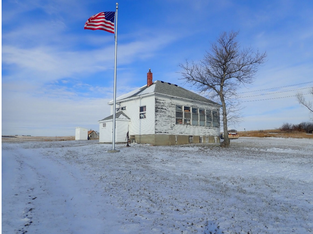
Figure 8: Feature 1, looking northwest.
