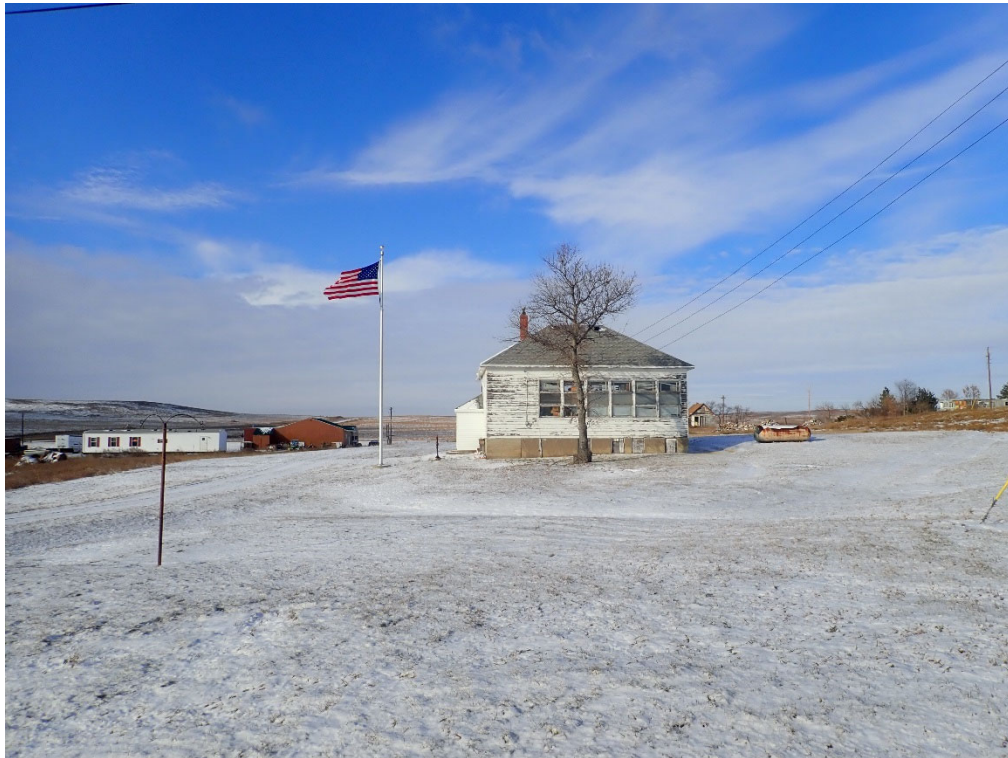
Figure 7: Feature 1, looking west.
