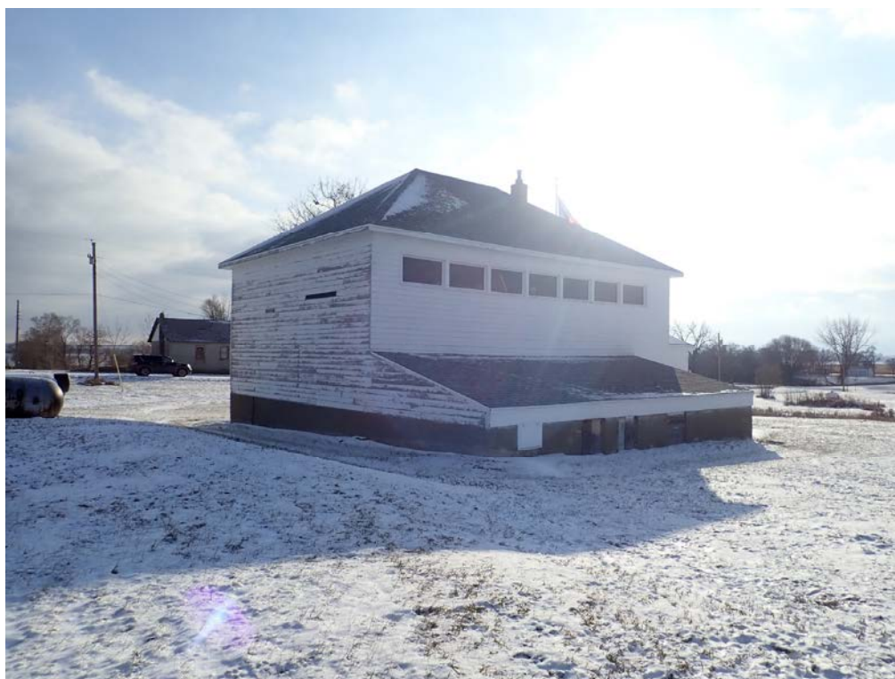
Figure 5: Feature 1, looking southeast, November 13, 2019.
