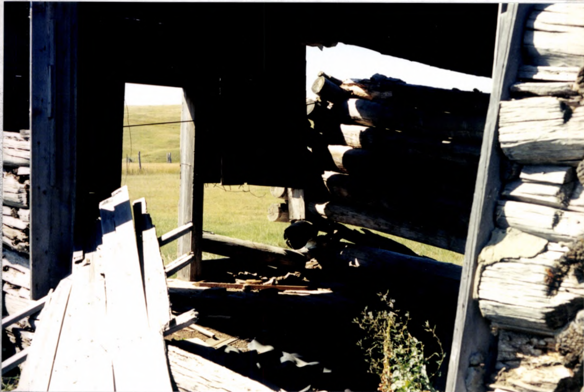
Interior SW From East Window
