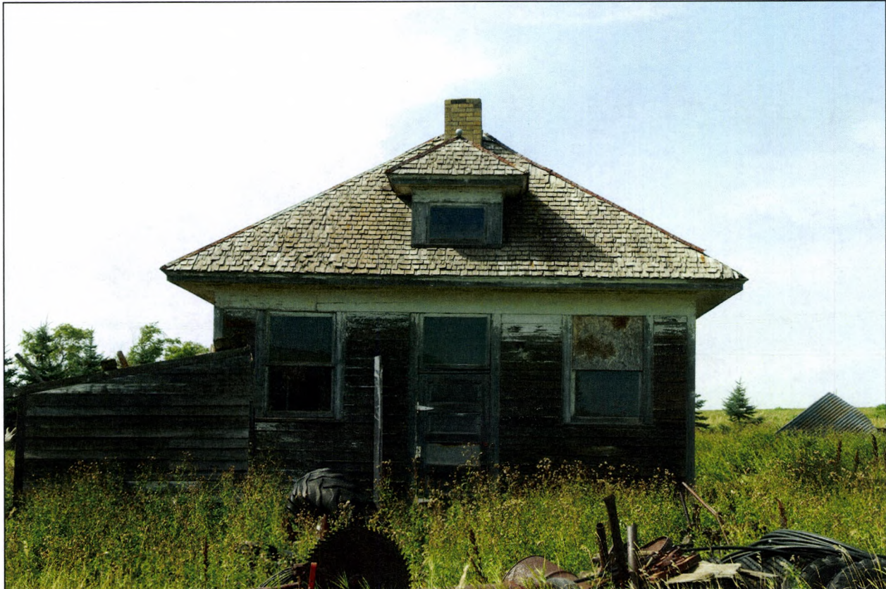
Figure 1. Rhoades School, east elevation (originally south).
