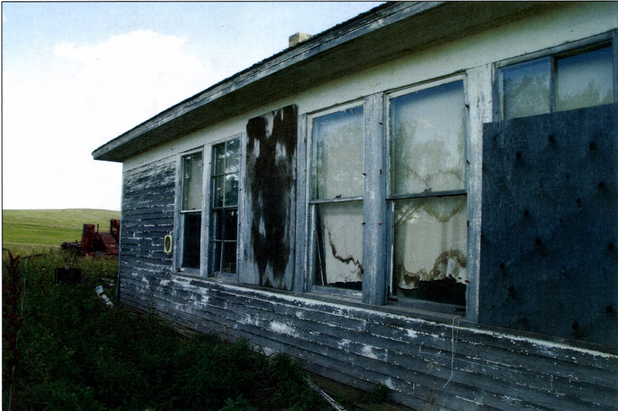
Figure 4. Rhoades School, north elevation (originally east).
