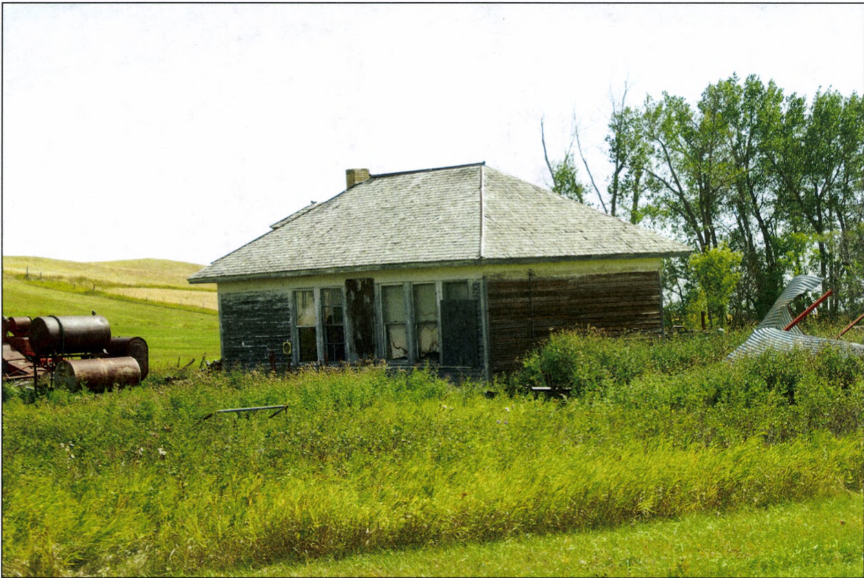
Figure 3. Rhoades School, north and west elevation (originally east and north).
