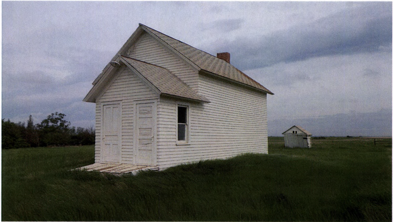
Figure 2: Overview of MAC-MNB-1009, view to the northwest (Image 3118).
